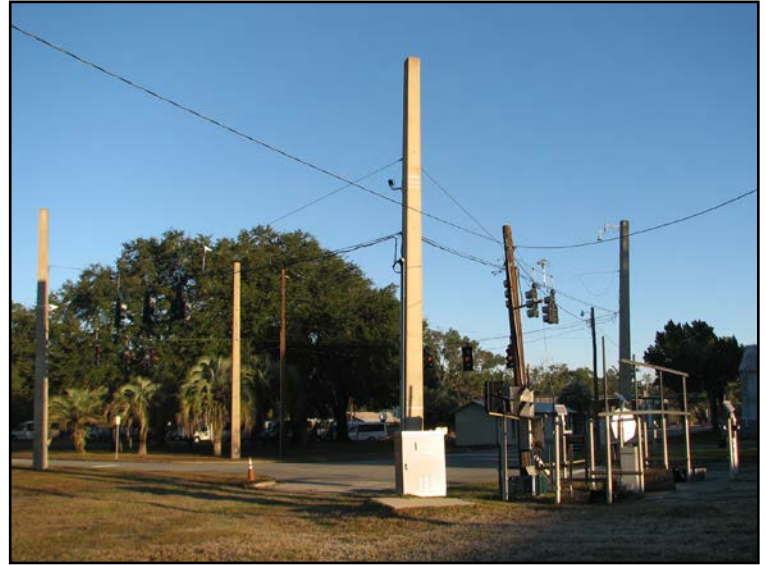
Older span wire intersection.
