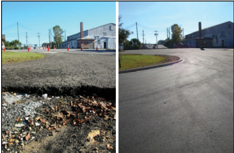
East/west connector intersection before and after.
