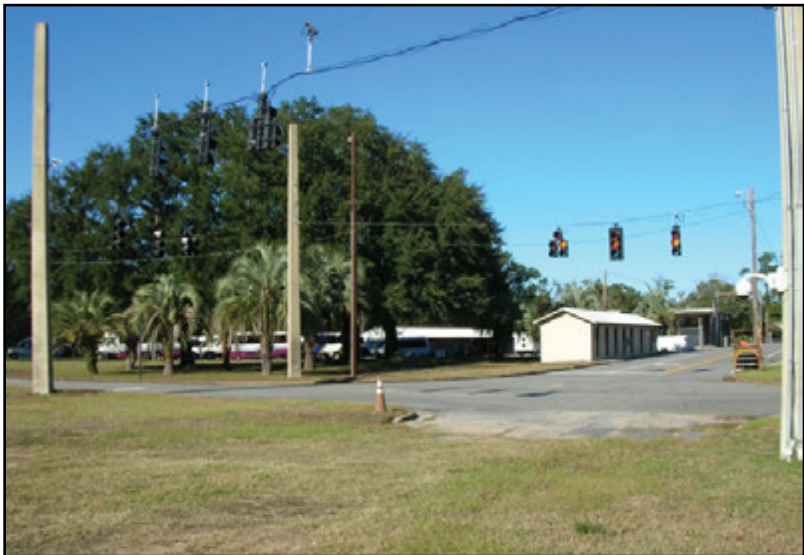
Realigned and extended span wire intersection. (Before - above; after - below)
