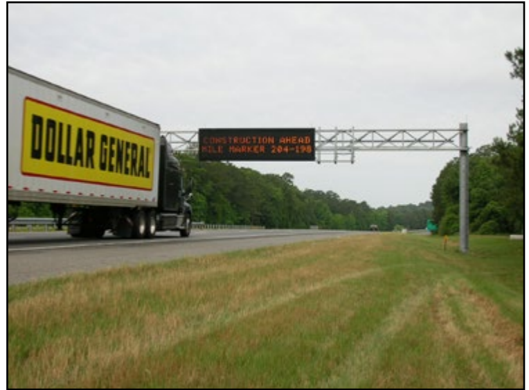
Existing DMS on I-10.
