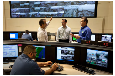
District Six TMC staff manage I-95 with several congestion management tools, such as ramp signaling.
