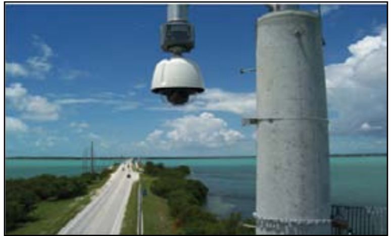
Closed-circuit television camera help with traffic management efforts in Monroe County.
