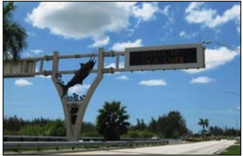
Dynamic message sign informs Monroe County travelers of real-time traffic conditions.
