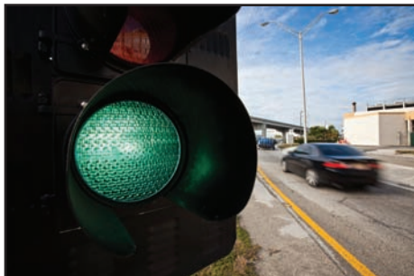
I-95 Ramp Signaling System is the first of its type in the state of Florida.
