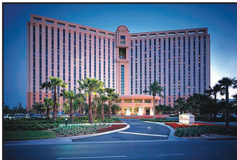
Rosen Centre in Orlando, Florida
