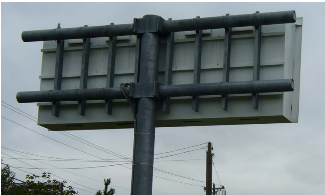
Figure A.3 – Back of a North Carolina DMS Structure
