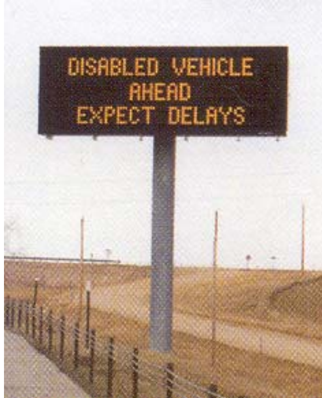
Figure A.4 – South Dakota DMS Structure i
