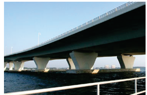
Post-tensioned concrete is critical to many kinds of construction, such as this box girder bridge.
