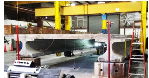
The full-scale test setup with simulated widening edge on the right is shown.
