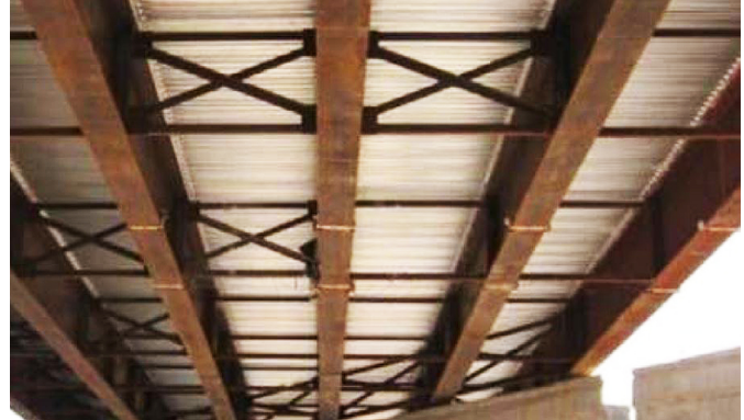
Cross-bracing system installed on a skew bridge.
