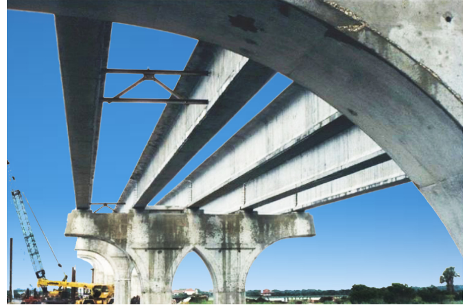
Cross-bracing between bridge girders.
