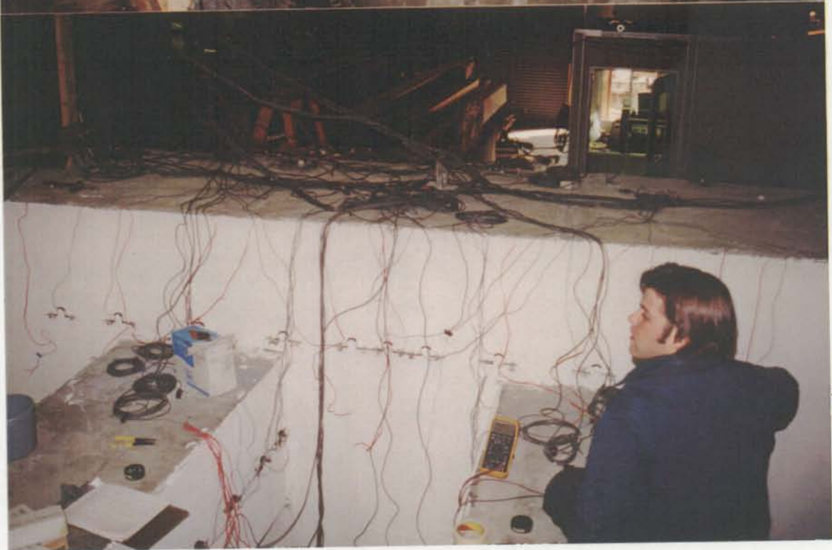
-Strip the Form from the Pile Cap Test Specimen. -Instrumentation of the Test Specimen.
