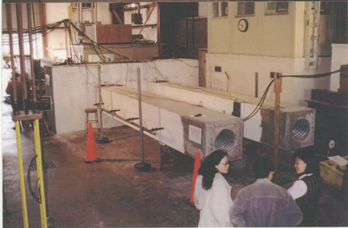
-Test Setup with the 30" PC Piles Embedded 48" in the Pile Cap and extended 21 ft. from the face of the Pile Cap.
