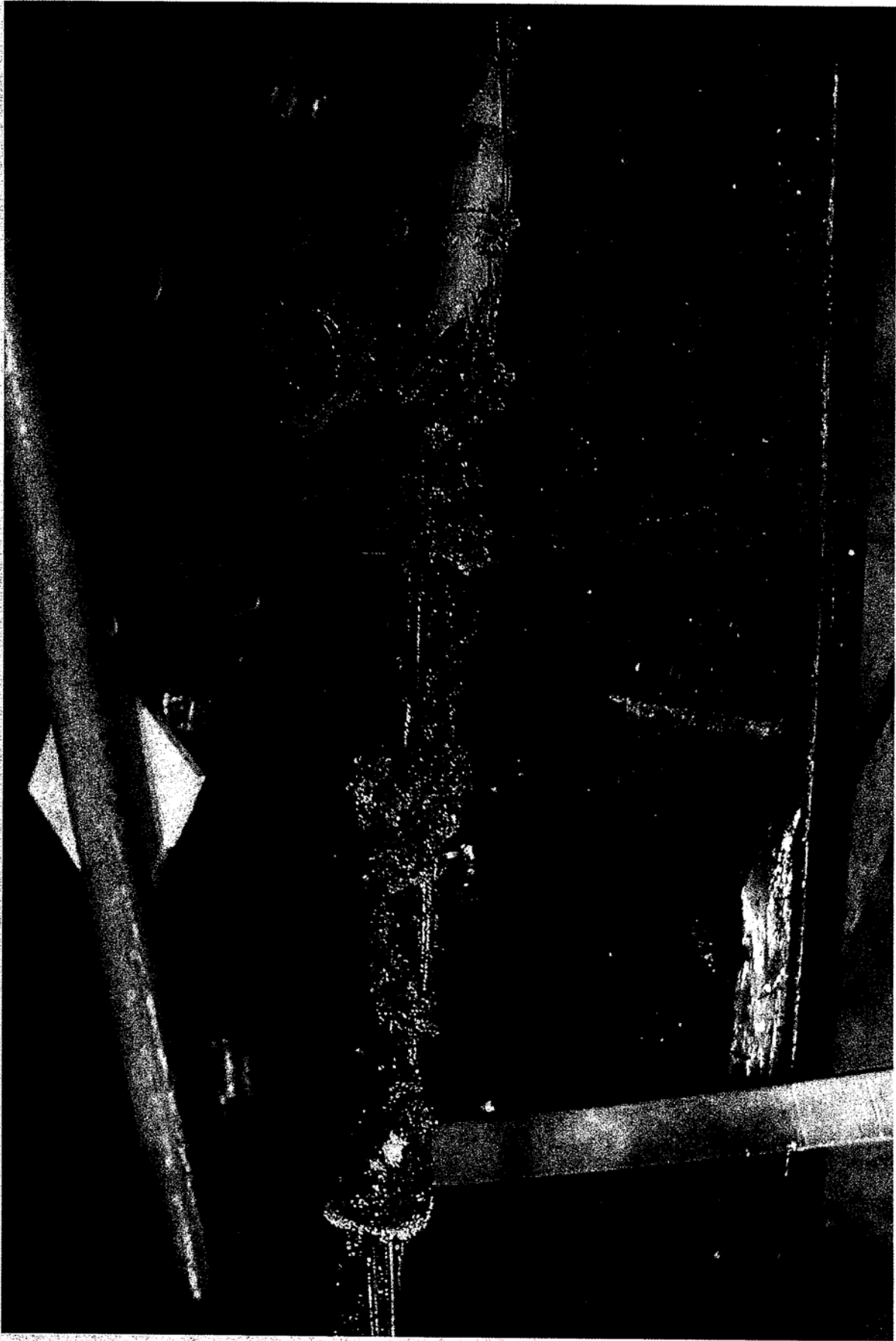
STRAND AFTER PVC PIPE REMOVAL
