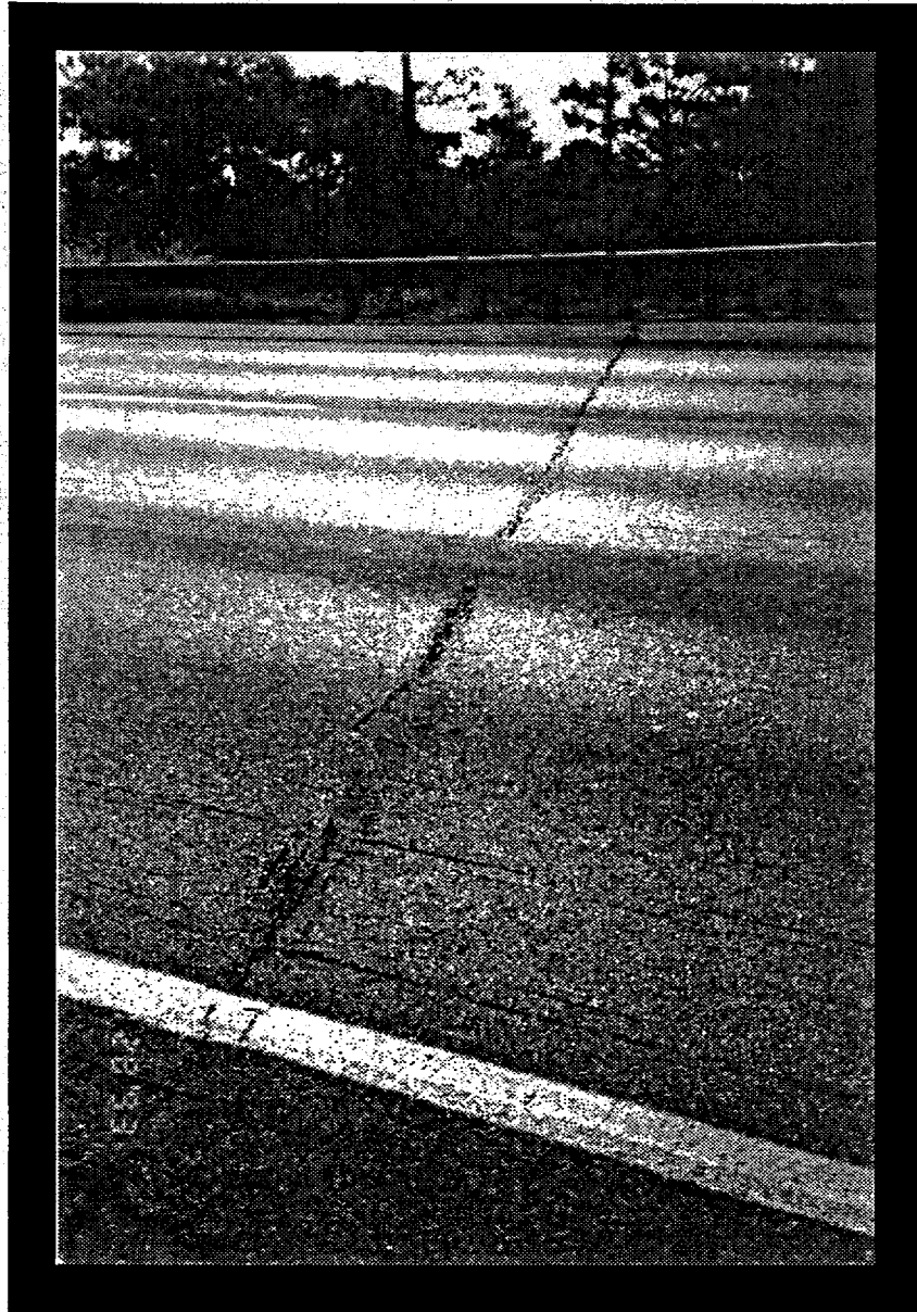
Koch BJS Joint System: Roadway Prior to Installation of Joint System
