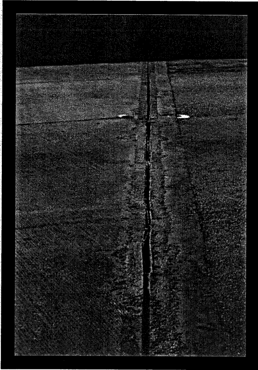
Polymer Concrete Inc.: RESURF IV (Replaced Nosing)
