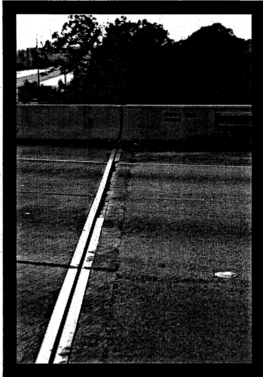
Problem Armored Joint on I-95: Missing Angle & Broken Concrete
