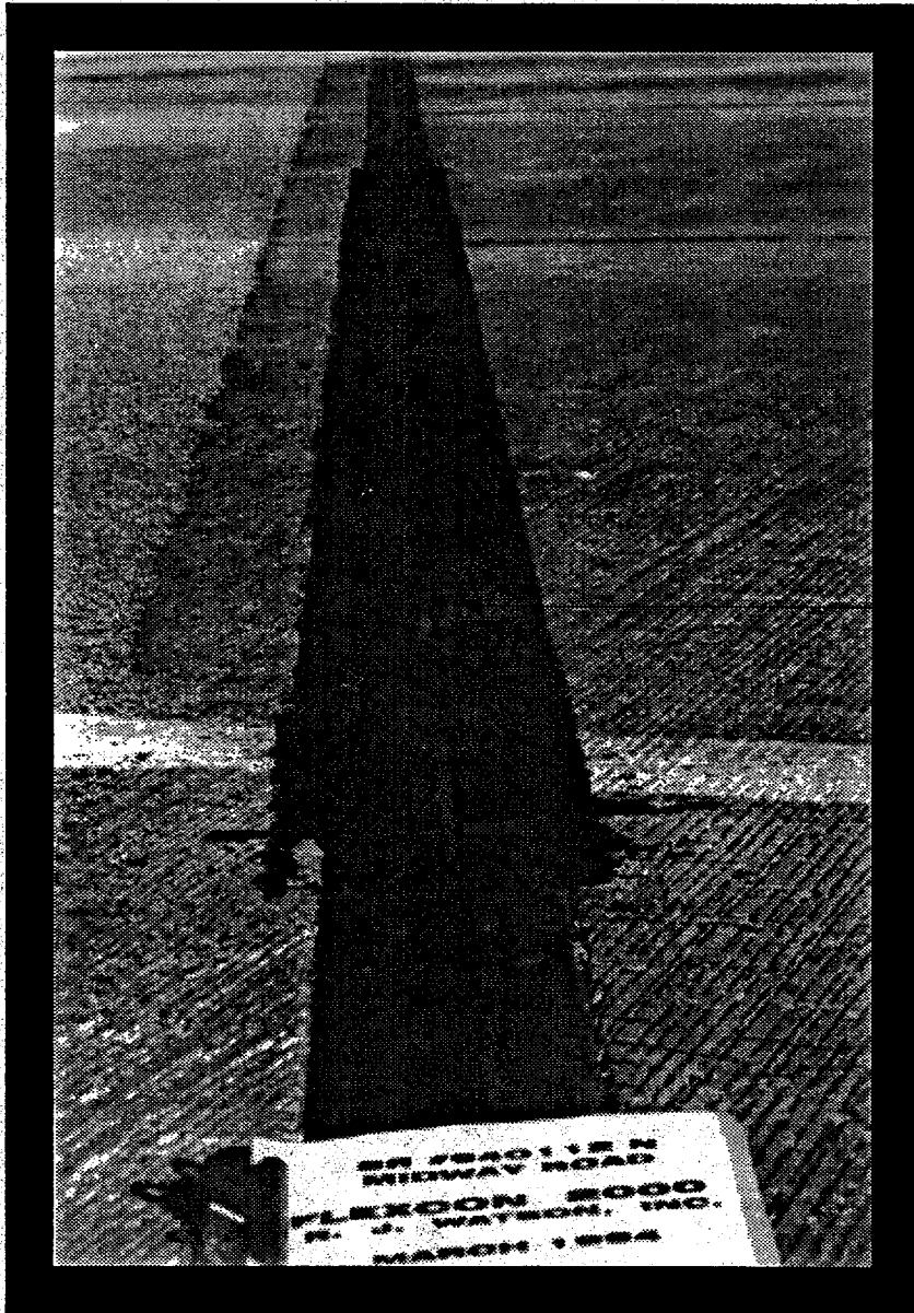
R. J. Watson: Flexcon 2000 Joint Sealing System (Problem Area)
