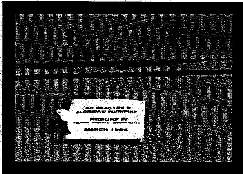
Polymer Concrete Inc.: RESURF IV (Failed Section)
