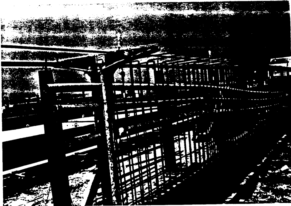
Figure 4.12 Interior Section of a Bulb-T Girder Before Casting
