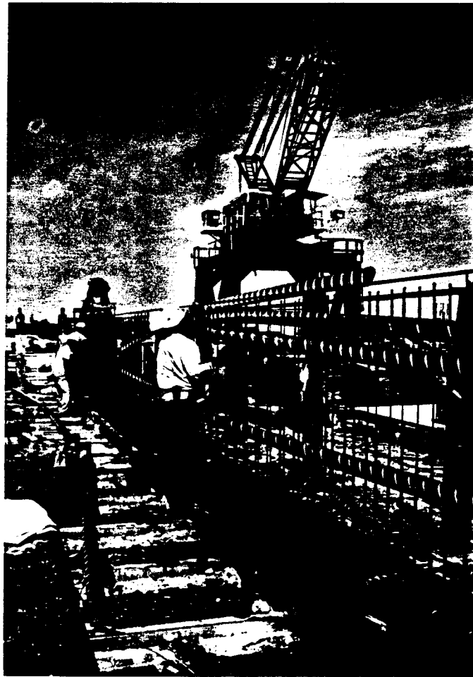
Figure 4.11 Placement of Oval Ducts in Bulb-T test Girder
