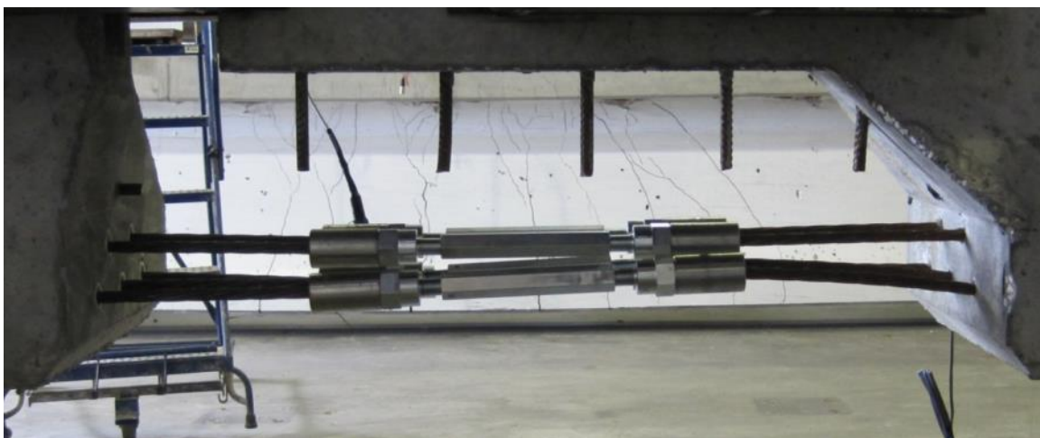
Figure 49–Coupled strand prior to prestressing
