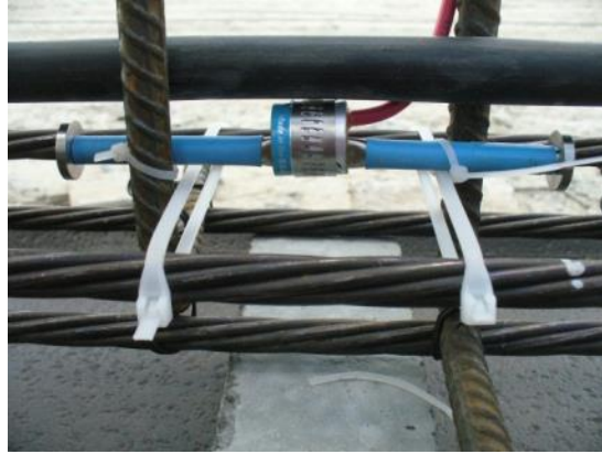
Figure 67–VWSG installation near centroid of strand pattern
