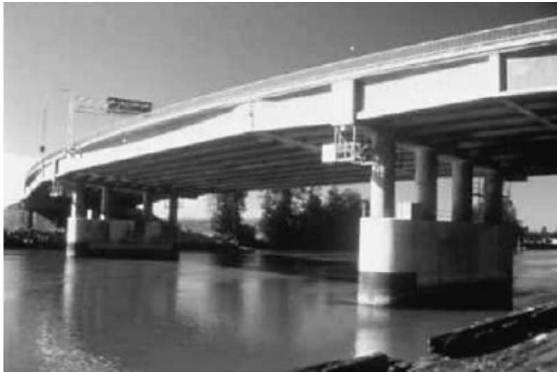
Figure 2–Curved roadway constructed with spliced girders (Abdel-Karim and Tadros 1992b)
