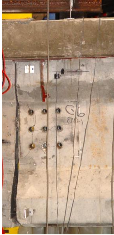
Figure 111-X1: Opening at joint during test
