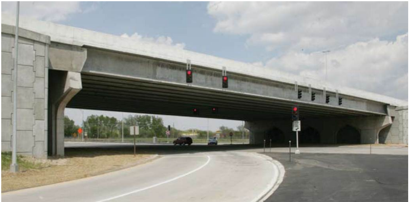
Figure 12–204th Street Bridge (Jaber et al. 2006)
