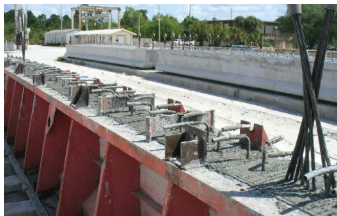
Figure 45–Segments after concrete is cast with top roughened for deck placement
