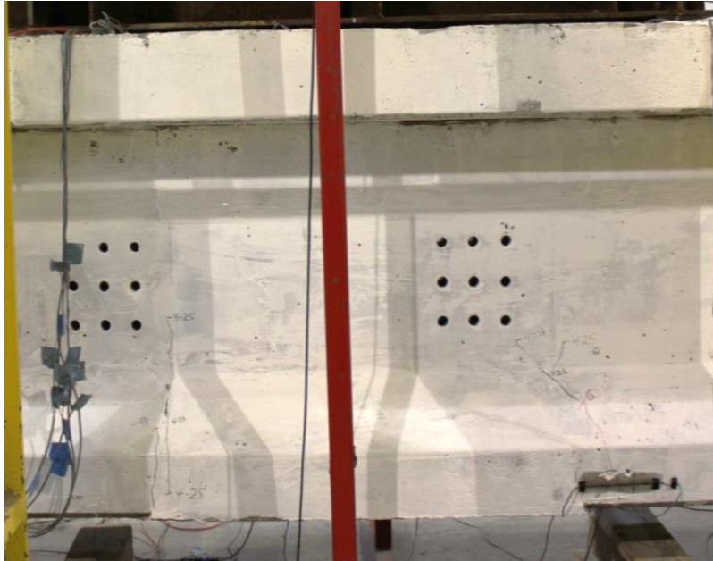
Figure 173–F2: Cracking after 2 million cycles
