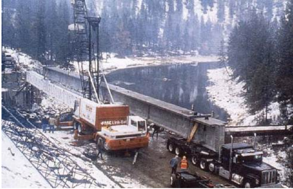
Figure 9—Launching assembled girder using trolley (Nicholls and Prussack 1997)
