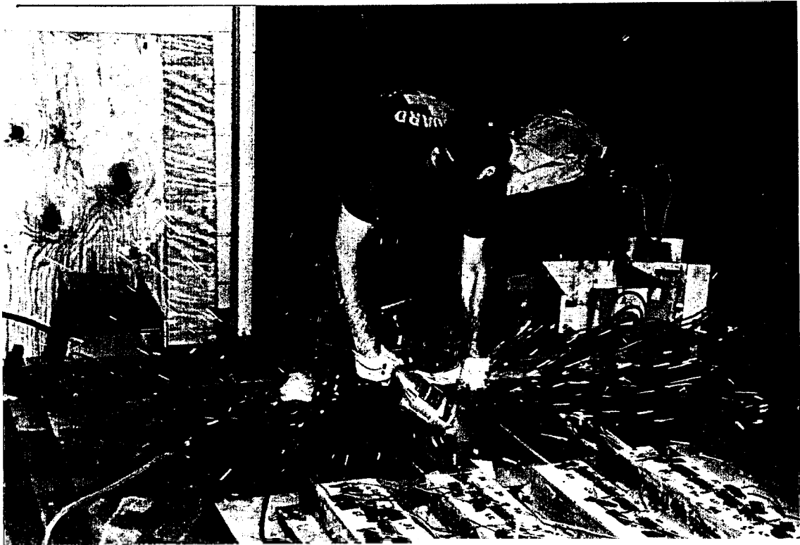
Plate 4.4 (top) Curing of specimens (btm) Release of prestressing force
