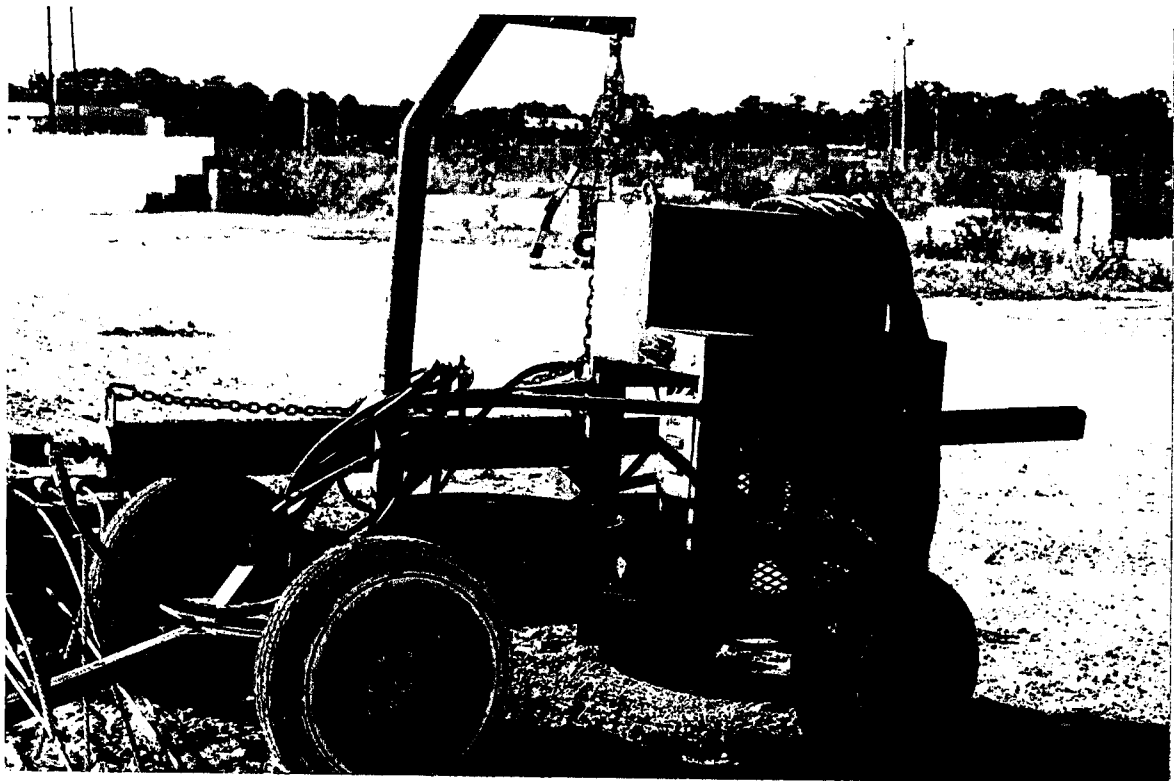
Plate 4.9 (top) Load cells at jacking end (btm) Prestressing jack used
