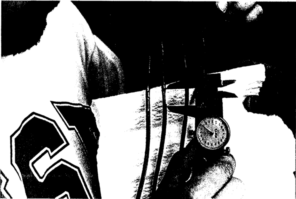
Plate 17.2 (top) Carbonation tests on ST-M2 (btm) Metal loss in steel strand in ST-M3
