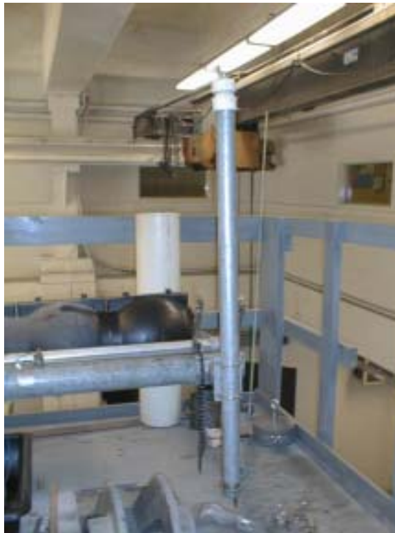
Figure 3.21 - 2 in Galvanized Pipe, Bungee and Mass Damper
