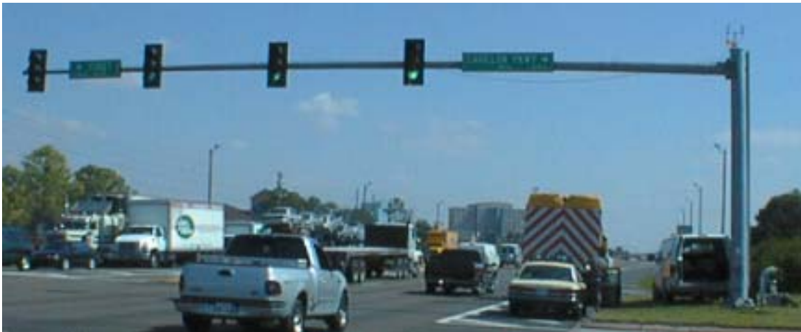
Figure 5.6 - Tampa Mast Arm
