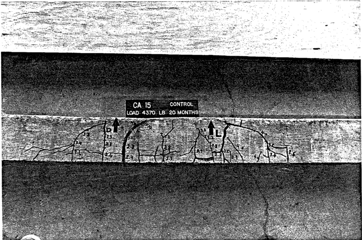
Plate 19. Crack Pattern of CA 15 - 20 Months
