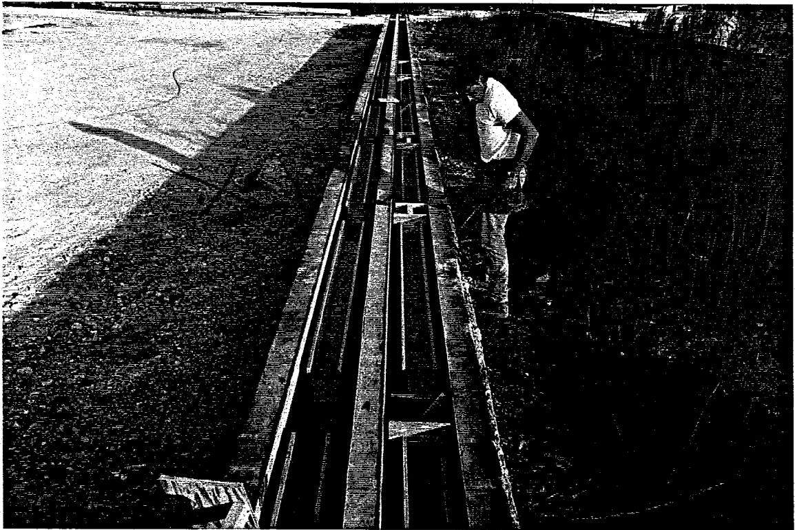
Plate 2. Prestressing Bed with All Thirty Three Forms
