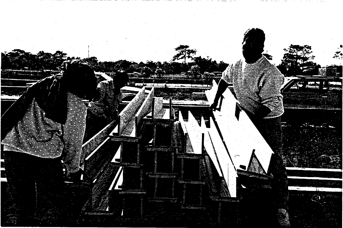
Plate 1. Installation of Formwork
