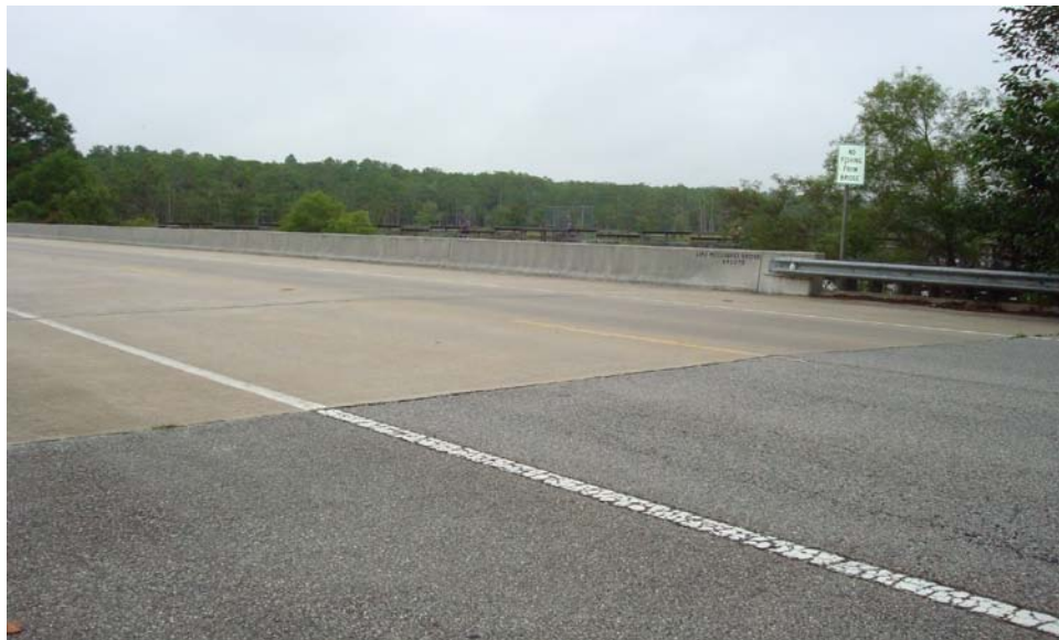
Figure 4.3. An abutment joint of bridge #540072
