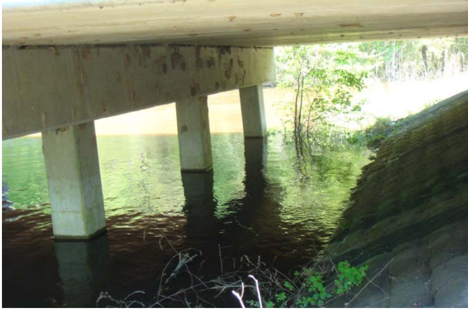
Figure 4.9. A view under bridge #540061
