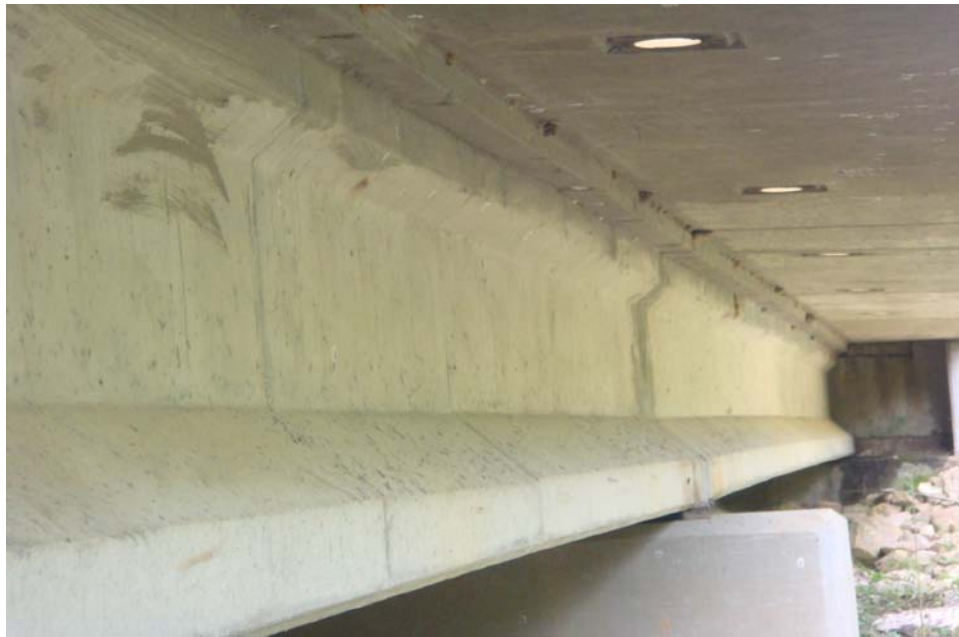
Figure 4.7. AASHTO type II girders of bridge #540074
