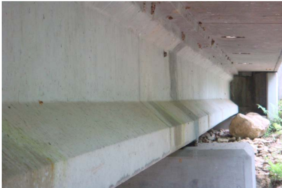
Figure 4.5. A view under bridge #540073
