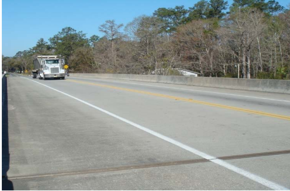
Figure 4.10. An approach of bridge #590056
