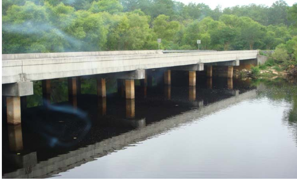
Figure 4.2. A side view of bridge #540072
