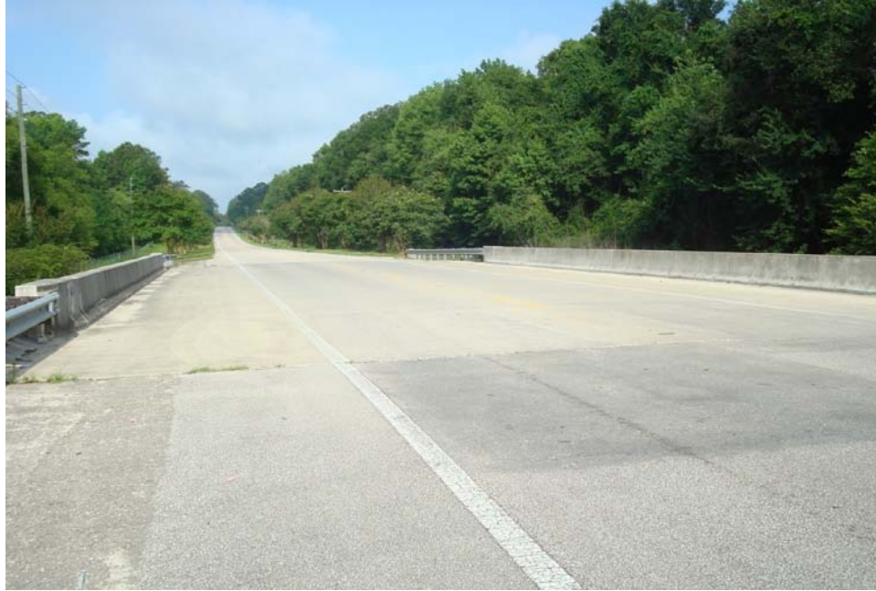
Figure 4.6. An approach of bridge #540074
