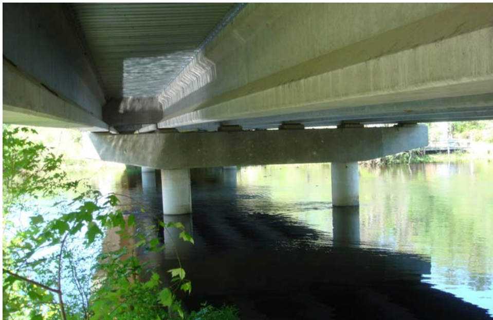
Figure 4.11. A view under bridge #590056
