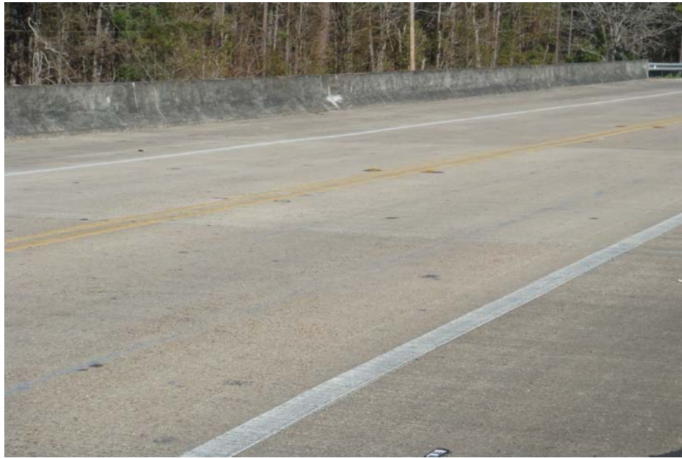
Figure 4.8. An approach of bridge #540061
