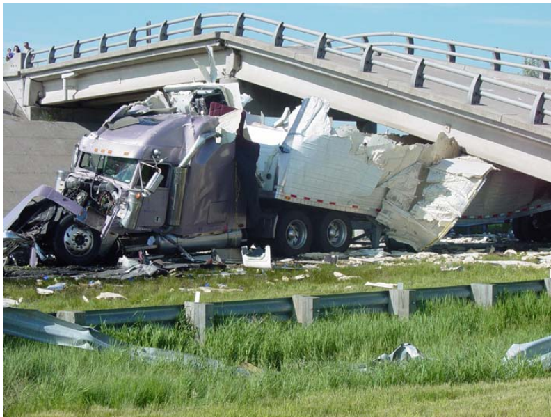
Figure 9.2. An example of the extensive damage resulting from an accident on I-80
