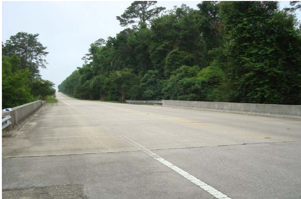
Figure 4.4. An approach of bridge #540073
