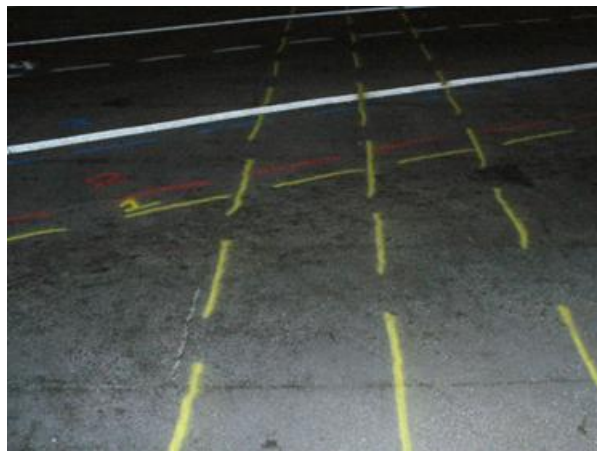
Figure 43 – Truck position reference marks on the bridge deck
