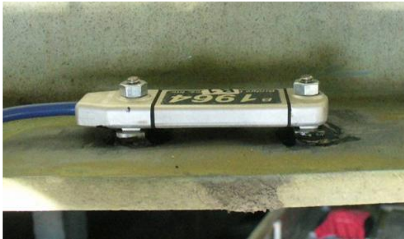
Figure 22 – Installed FBS gage on the steel girder
