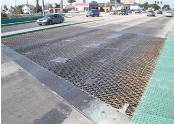
Figure 10 – Existing steel grid deck
