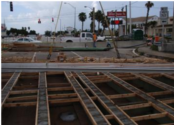
Figure 12 – Installation of bottom GFRP panels
