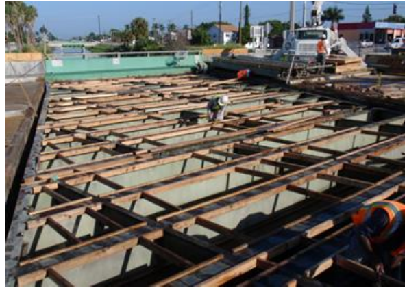
Figure 11 – Formwork for grout pads
