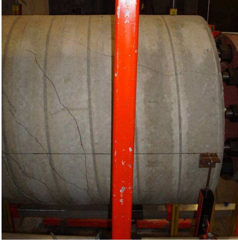
Figure 5-9. Torsional and flexural cracks forming
