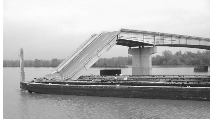
In 2003, a barge tow struck a pier of the I-40 bridge near Webbers Falls, Oklahoma. A portion of the superstructure collapsed and 14 people were killed.
