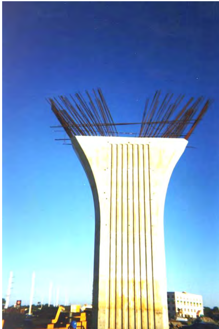
Figure 6-21: Pier Segment of the Roosevelt Bridge
