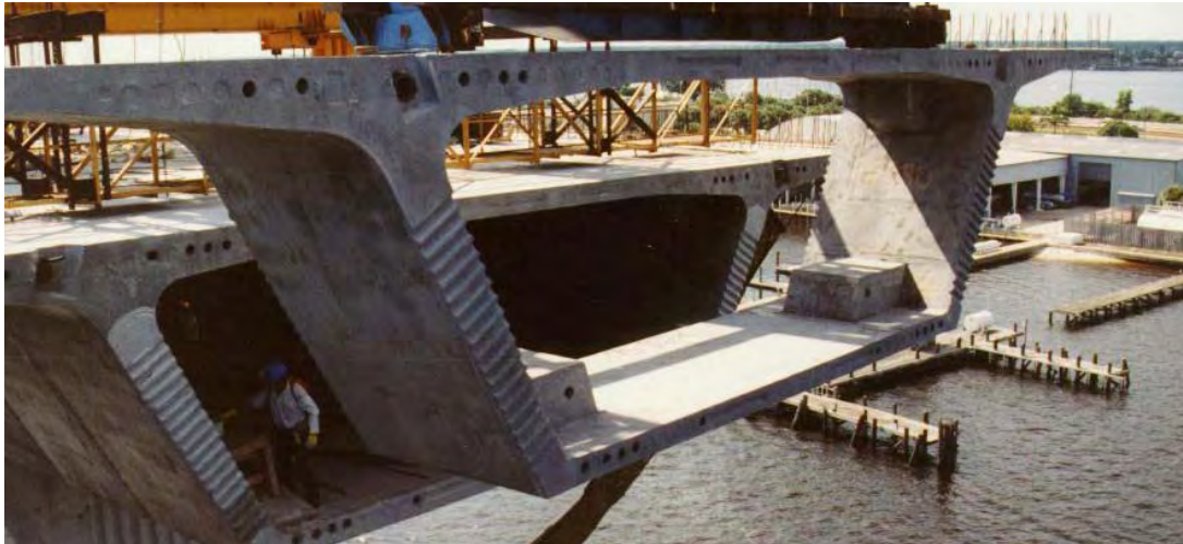
Figure 1-2: Segmental Box Girders
