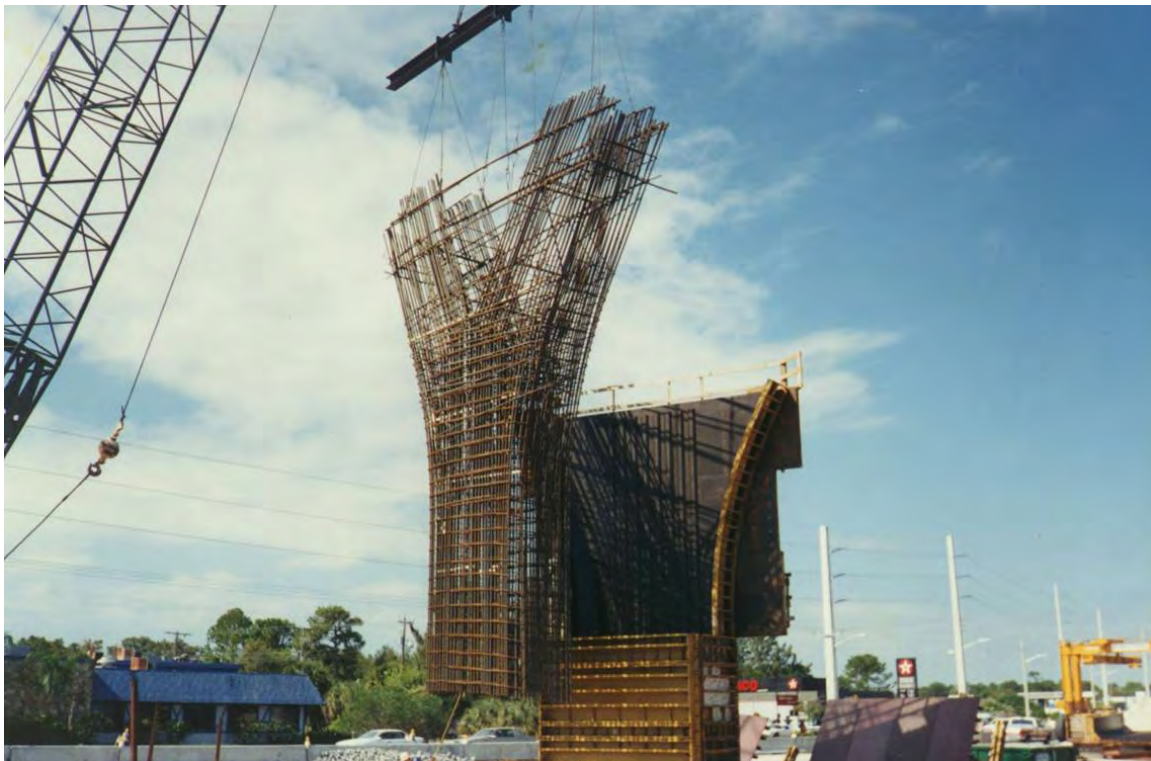
Figure 6-24: Reinforcing Steel Cage for A Pier Segment of the Roosevelt Bridge
