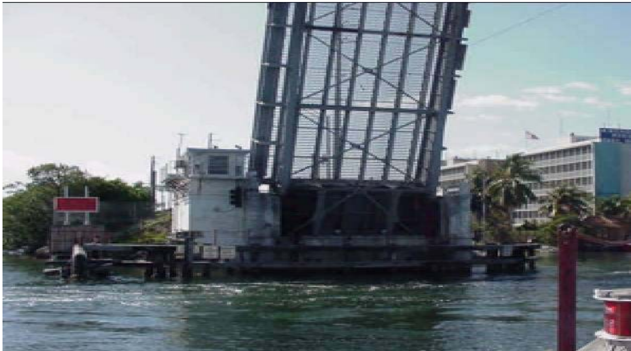
Figure 2-2: Open Steel Grate Deck Systems - Jewfish Creek Bascule Bridge.
