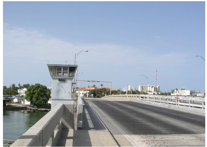
Typical steel grate bascule bridge
