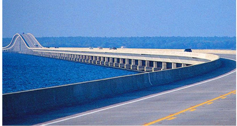
Building bridges like the 3.6-mile-long Mid-Bay Bridge in Okaloosa County depends on the design flexibility offered by post-tensioning technology.
