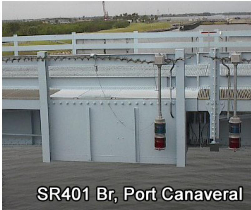
Figure 5.24 – Span lock
