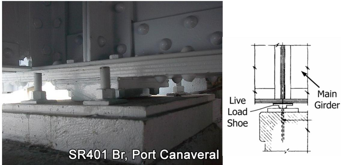
Figure 5.23 – Live load shoe (LLS) (sketch adapted from Christa McAuliffe Bridge construction plans)
