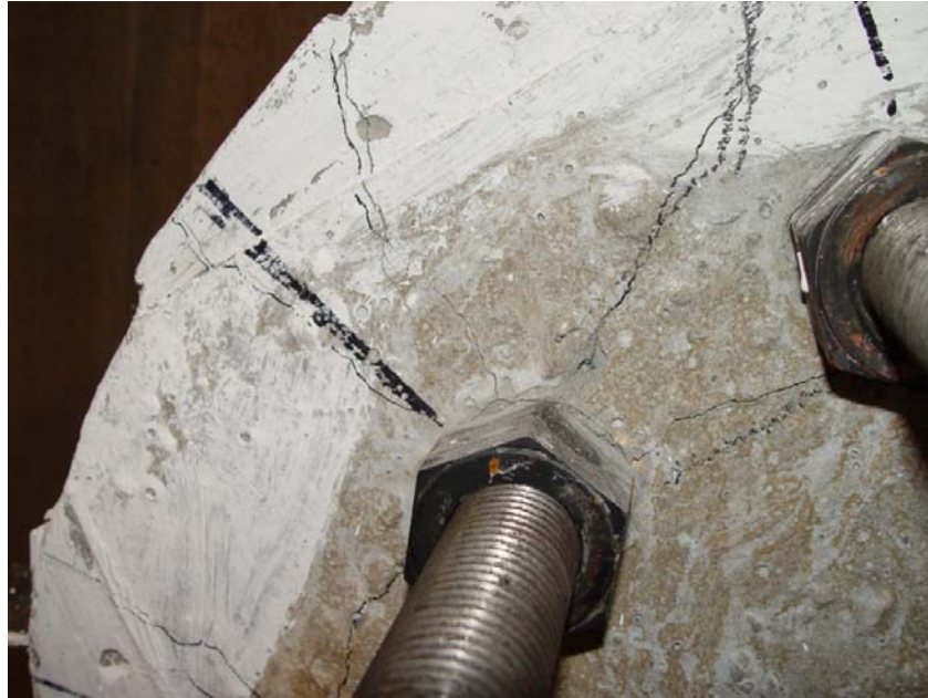
Figure 5-3. Face of test specimen after testing exhibits cracks between the bolts along with the characteristic concrete breakout cracks
