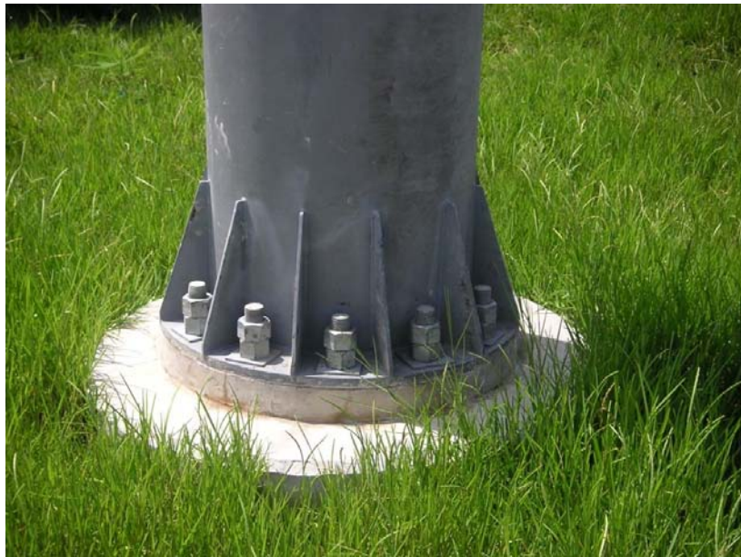
Figure 2-2. New foundation installed at the site
