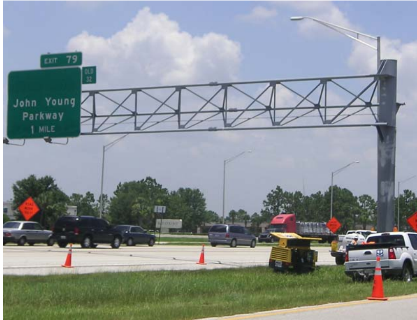
Figure 2-1. Cantilever sign structure at Exit 79 on Interstate 4 in Orlando
