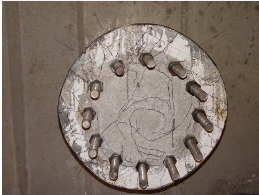
Figure 5-14. Face of shaft after test illustrates yielding of bolts, concrete breakout cracks around the perimeter, and torsion cracks in the center.
