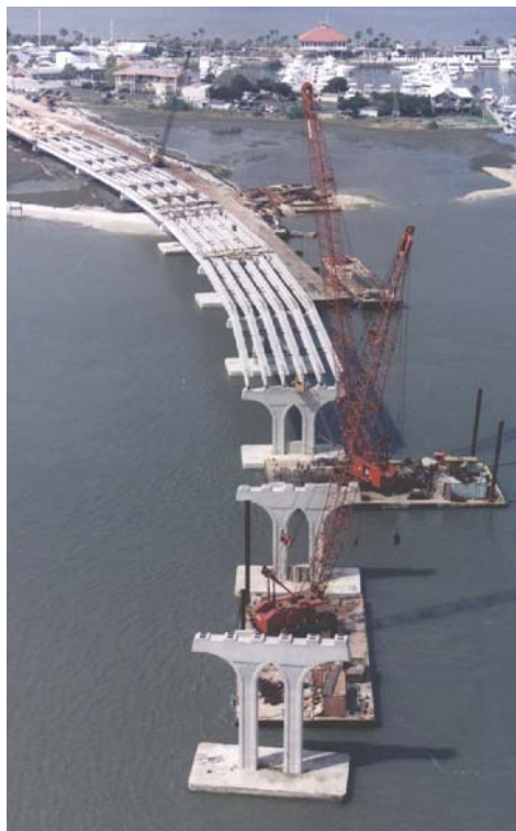
Figure 1.1 Construction of a girder-slab bridge using Florida bulb-tee girders (Vilano Beach Bridge, Florida / Photo credit: Florida DOT)
