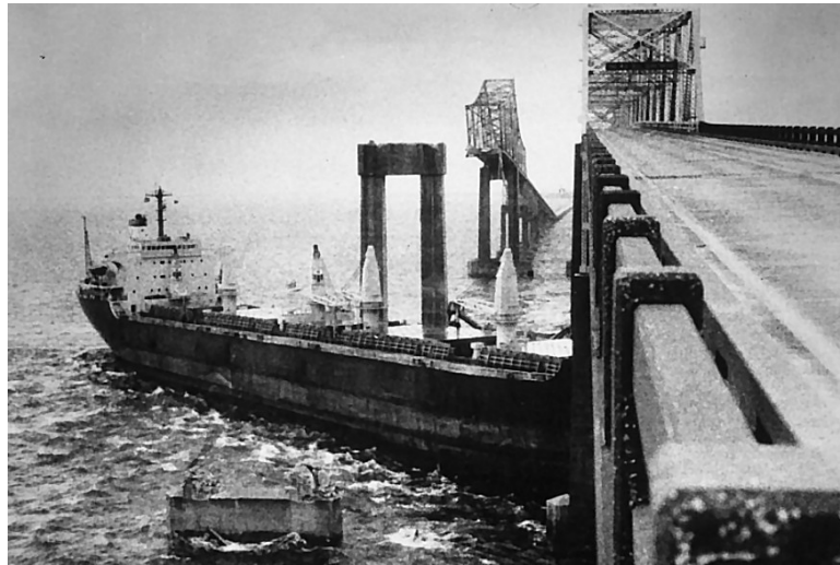
Figure 2.1 Collapse of the Sunshine Skyway Bridge in Florida (1980) after being struck by the cargo ship Summit Venture
