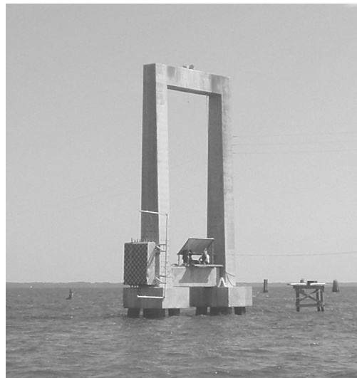
Figure 3.6 Pier-3 in isolation for the series P3 tests
