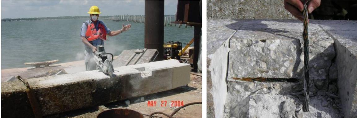
Figure 12 – Saw cut and strand removal
