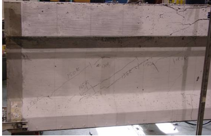
Figure 43. Failed SS2-STDF1 beam
