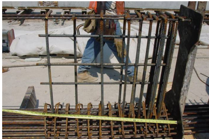
Figure 5. Stirrup and confinement reinforcement at end of non-capped shear beam
