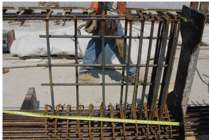
Figure 51. Stirrup and confinement reinforcement at end of non-capped shear beam
