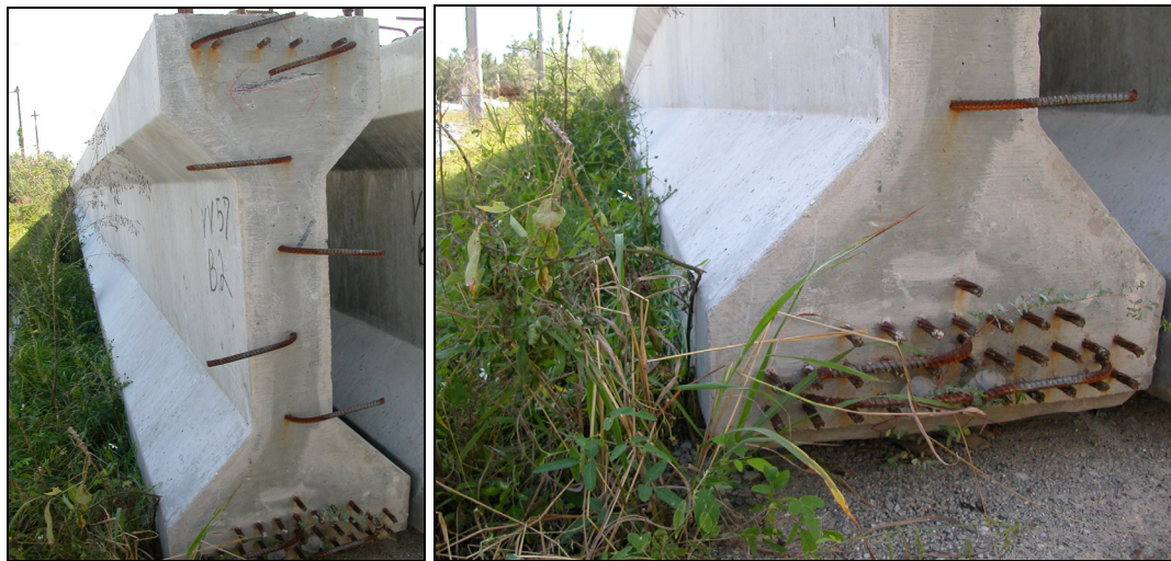
Figure 16. AASHTO Type IV girder in storage.
