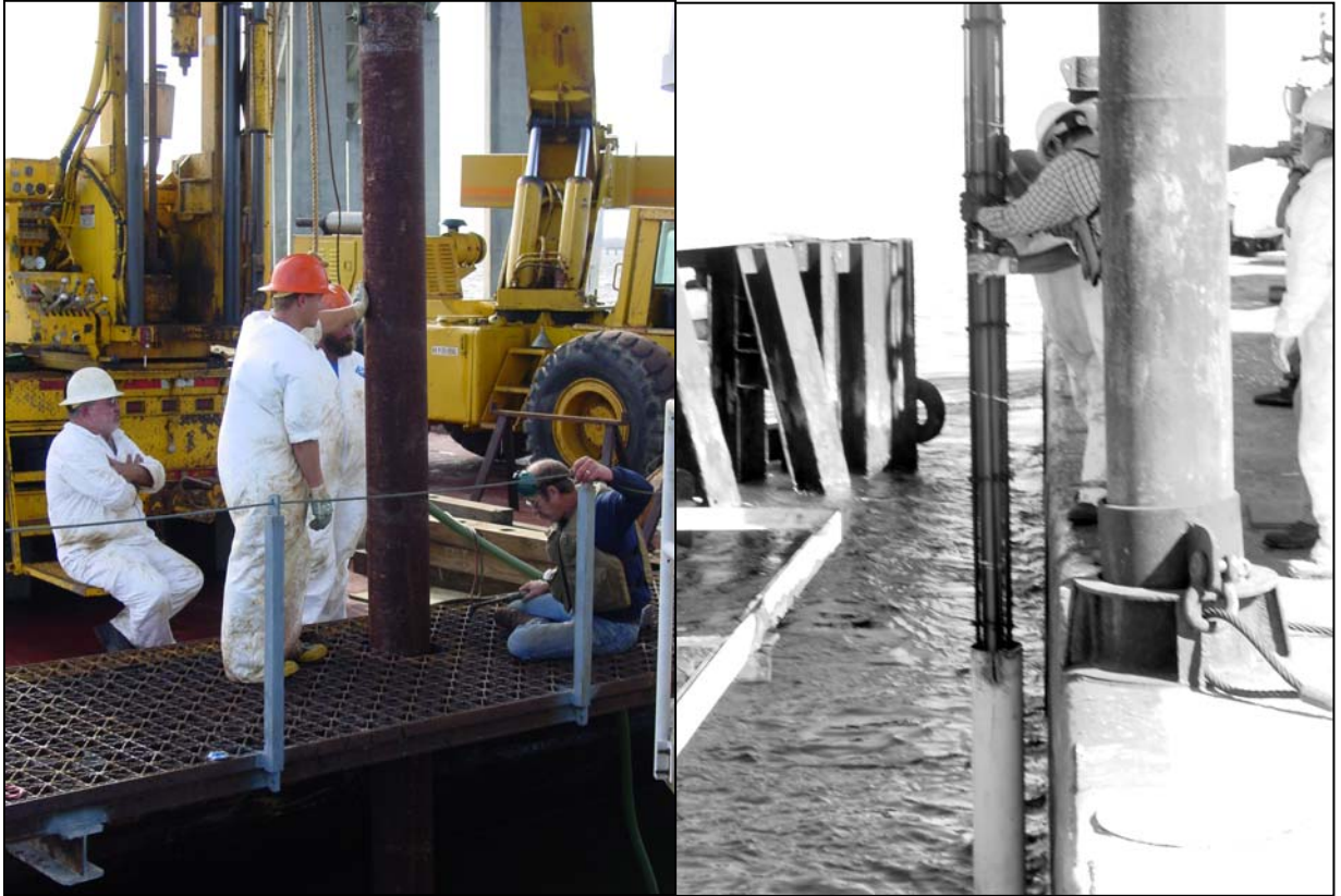
Figure 2.12 a) Placing ZW Casing
