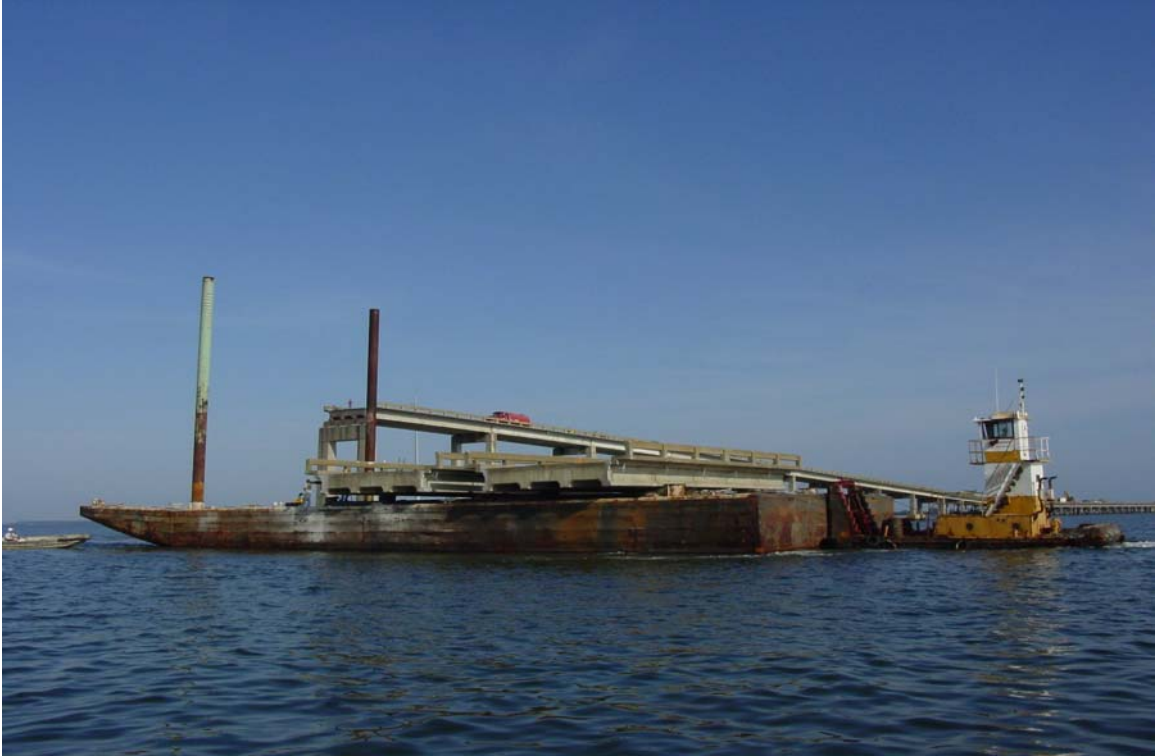
Figure 3.4 Deck Barge with Payload
