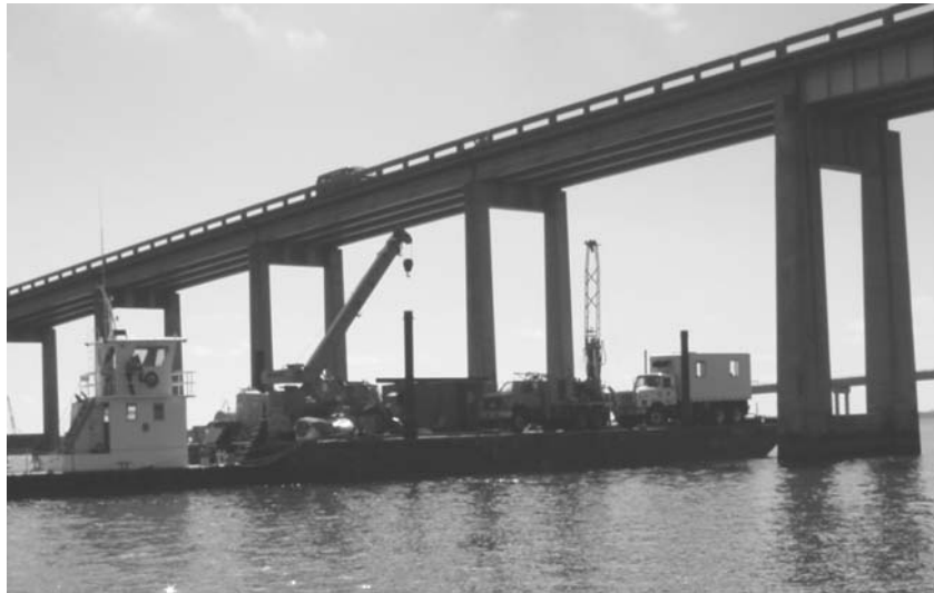
Figure 2.1 40 ft x 100 ft Spud Barge at Pier 3S
