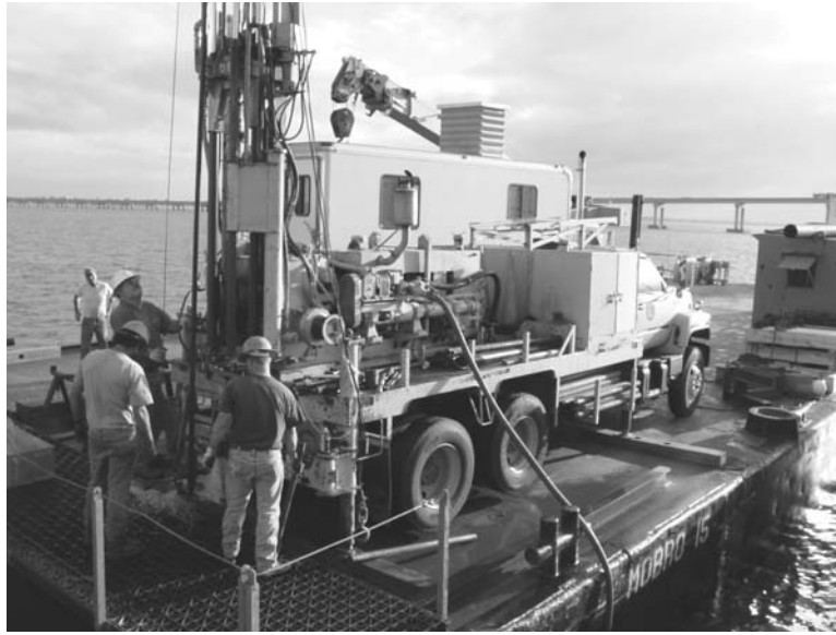
Figure 2.2 Drill Rig and CPT Rig at Pier 1S
