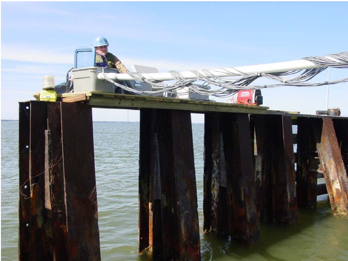
Figure 3.3 Fender System and Working Platform
