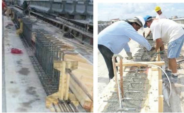
Figure 41. Girder construction.
