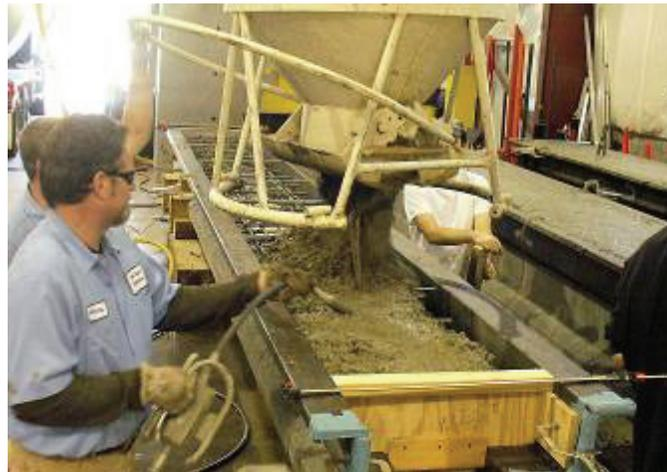
Figure 45. Deck concrete placement and vibration.
