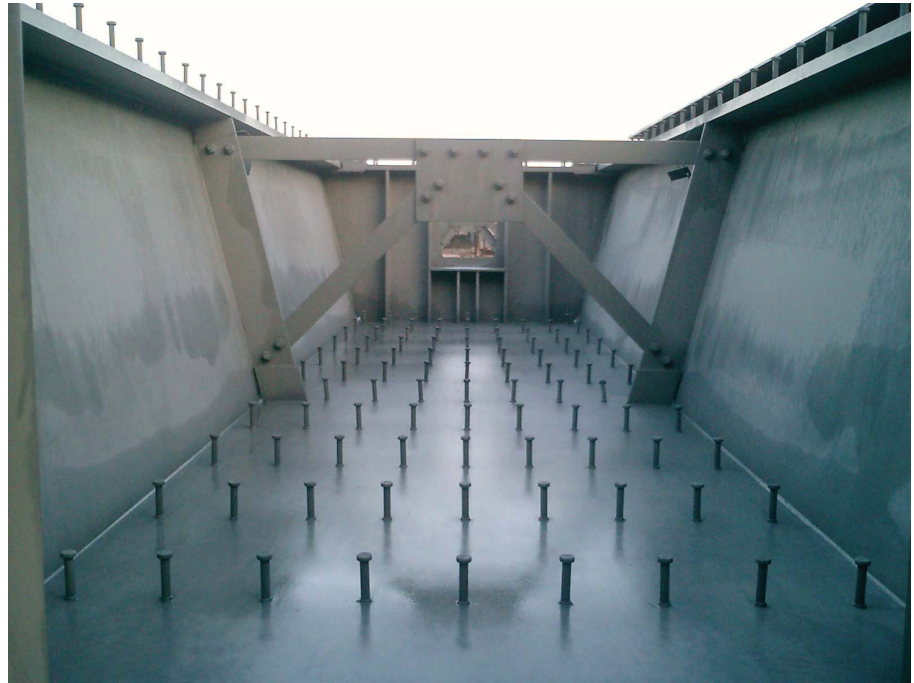
Double composite box girder
