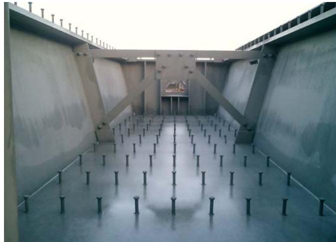
Figure 2.6 Shear Connectors and Interior Cross Frames
