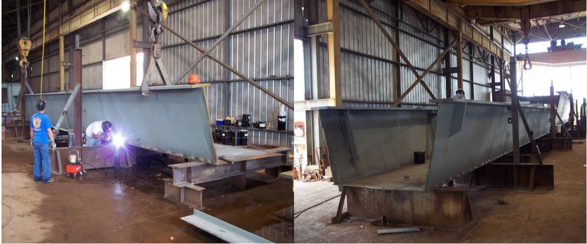
Figure 3.6 Assembly of Steel Box Section
