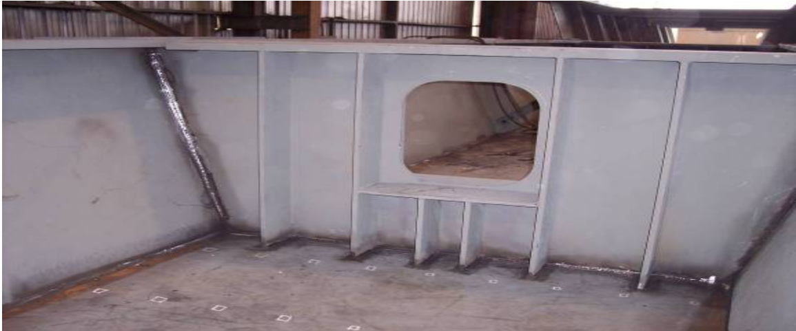
Figure 3.9 Diaphragm Welded to Steel Box
