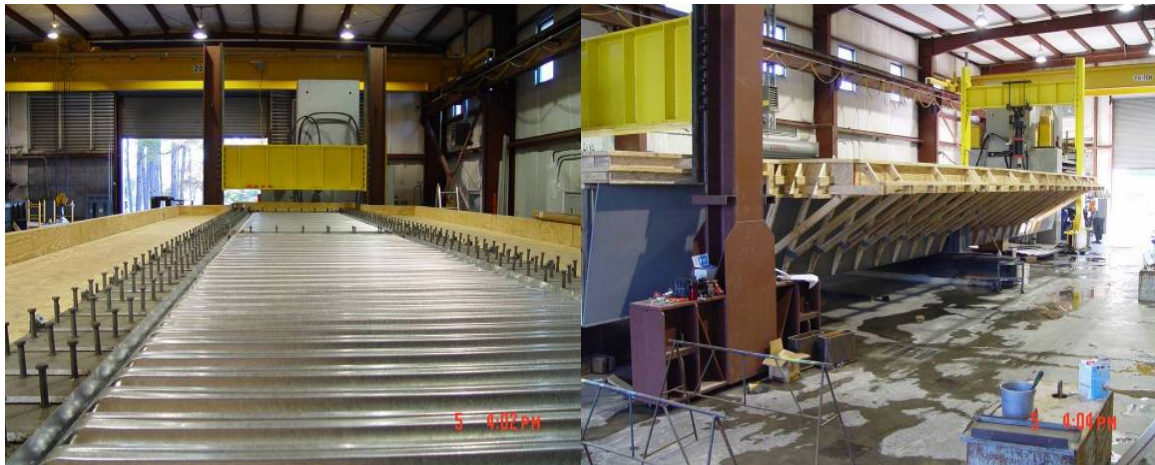
Figure 3.16 Stay in Place Forms and Overhang Brackets for Top Slab
