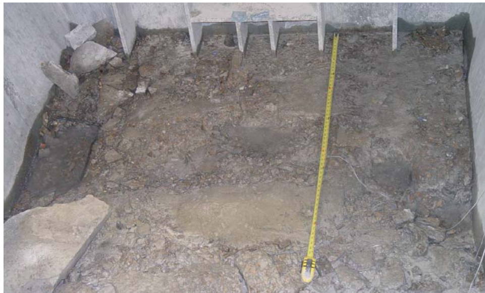
Figure 7.2 View of Bottom Slab on Hold Down Side After Clean-up
