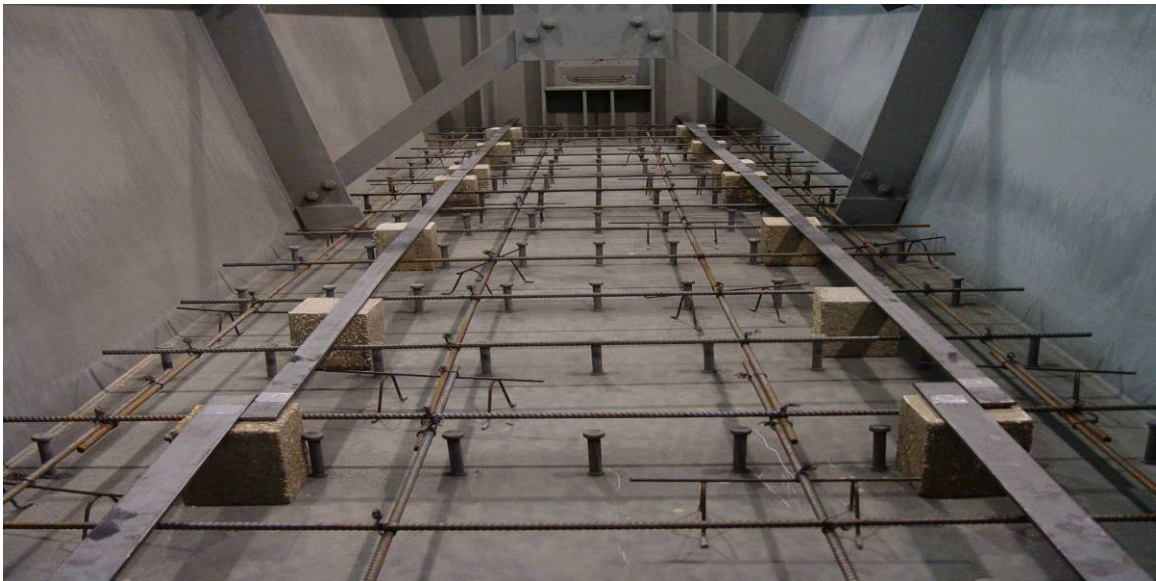
Figure 5.5 Placement of Bottom Concrete Slab
