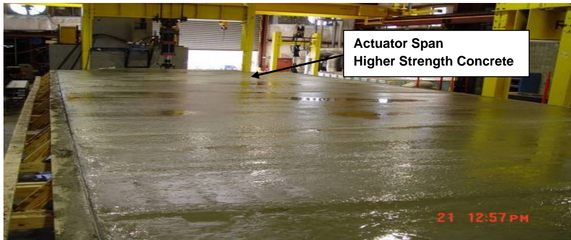
Figure 3.19 Top Concrete Slab
