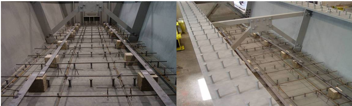
Figure 3.14 Reinforcement for Bottom Concrete Slab
