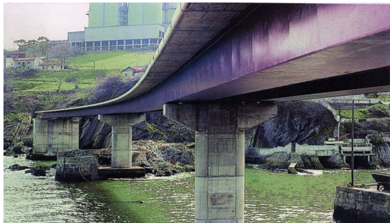
Figure 1.1 First Double Composite Bridge, Ciervana Bridge ( Courtesy J.M. Calzon )
