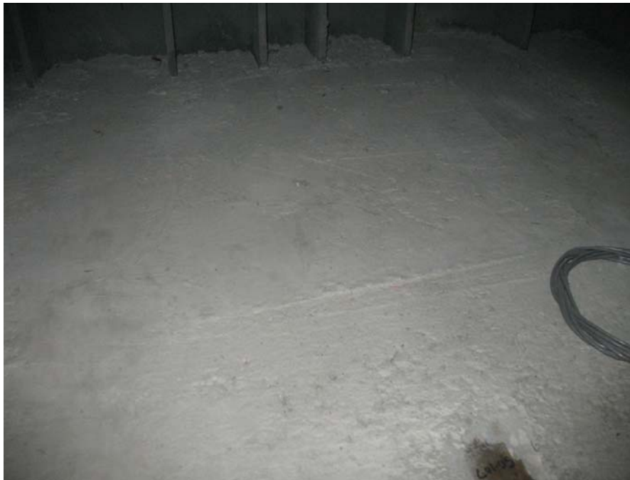
Figure 9.2 Bottom Slab on Actuator Side Showing No Signs of Deterioration
