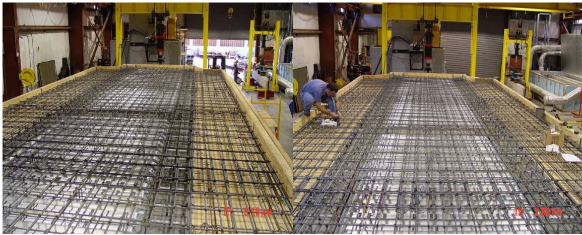
Figure 3.17 Reinforcement for Top Concrete Slab
