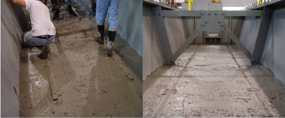
Figure 3.15 Pouring of Bottom Concrete Slab
