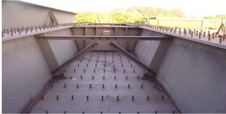
Figure 3.12 View of Shear Connectors Welded to the Bottom Flange
