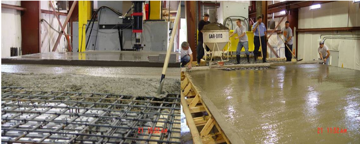
Figure 3.18 Pouring of Top Concrete Slab
