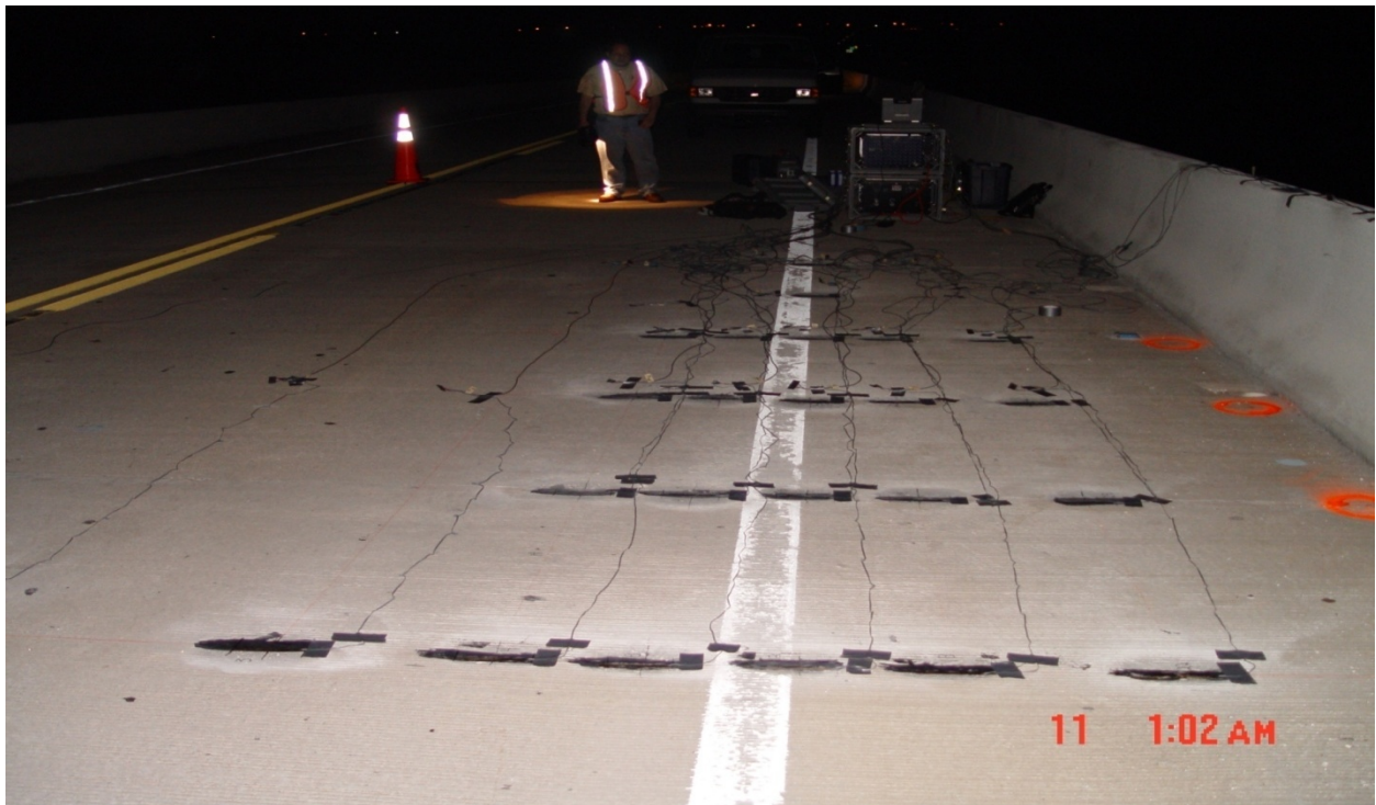
Figure 39: Channel Five Bridge Test Strain Gages.
