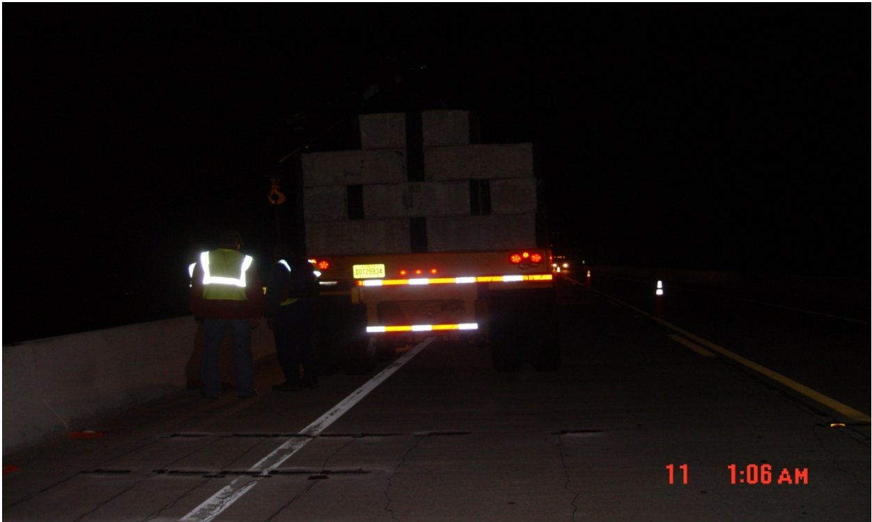
Figure 35: Channel Five Bridge Loading.
