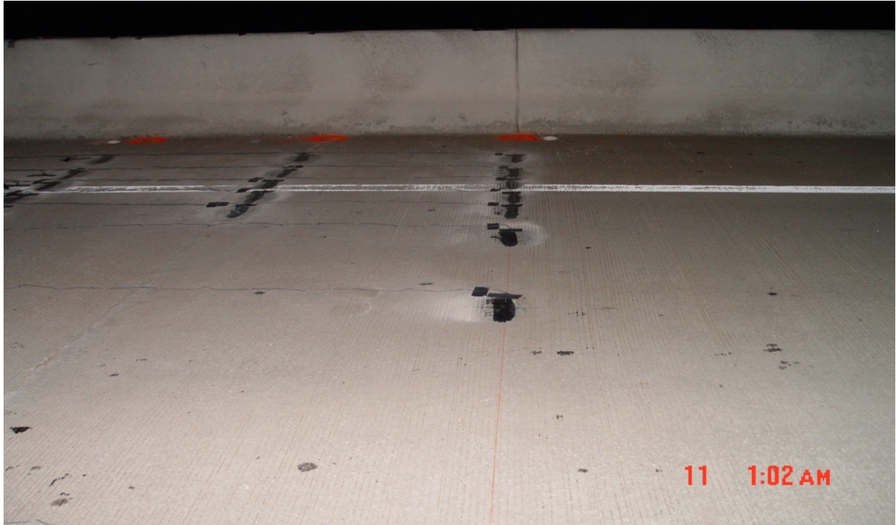
Figure 38: Channel Five Bridge Test Barrier Joint.
