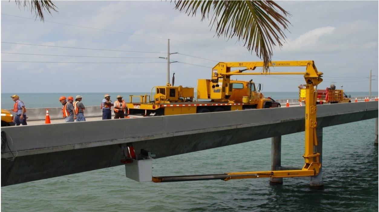
Figure 32: Gage Placement under the Seven Mile Bridge Deck with the Snooper.
