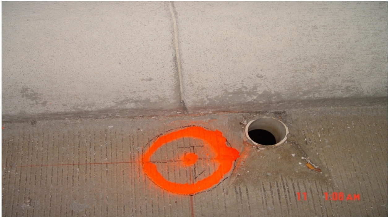
Figure 37: Channel Five Bridge Test Load Position 1 at the Barrier Joint.
