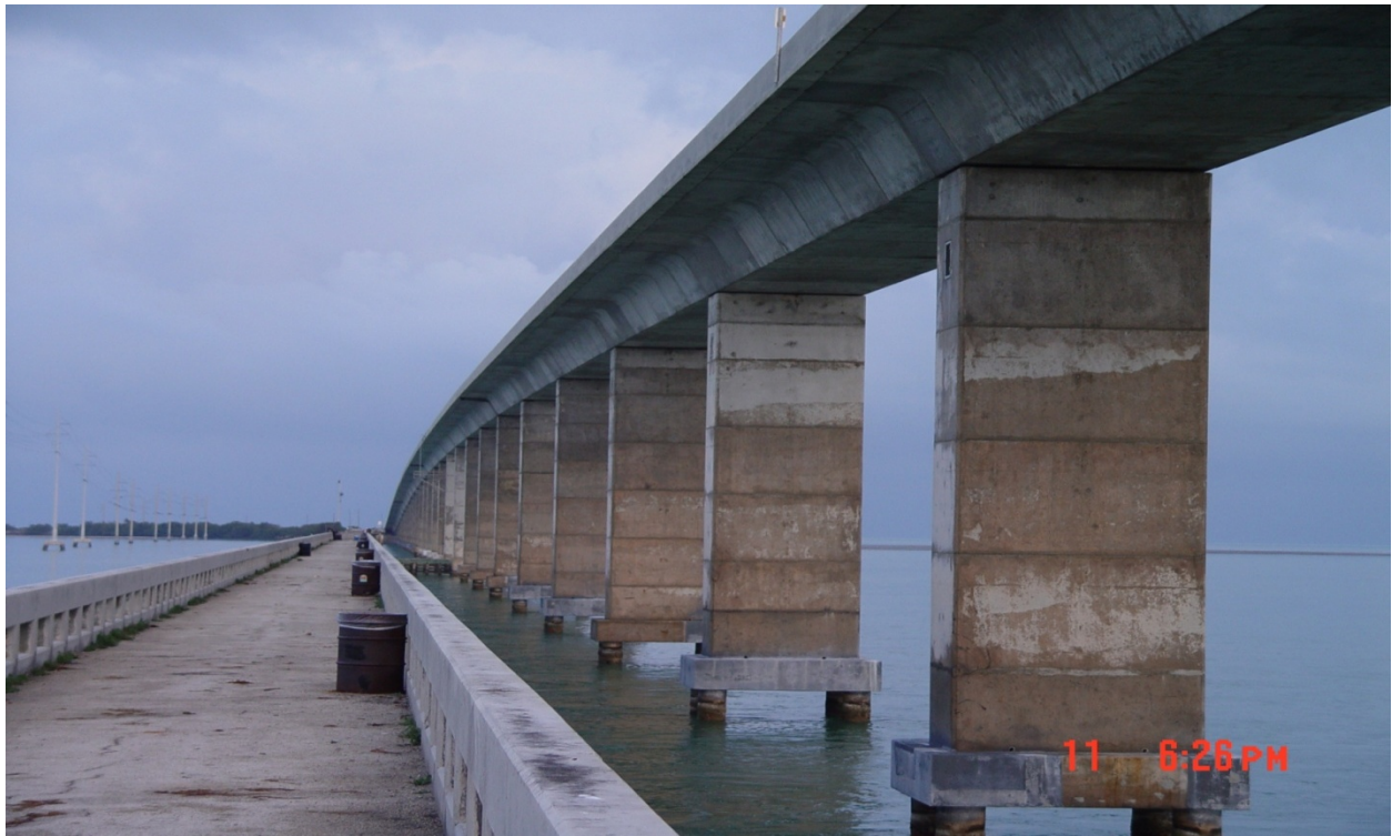
Figure 42: Channel Five Bridge.
