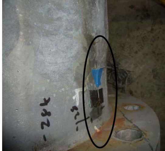
Figure 5. Strain Gage Installation
