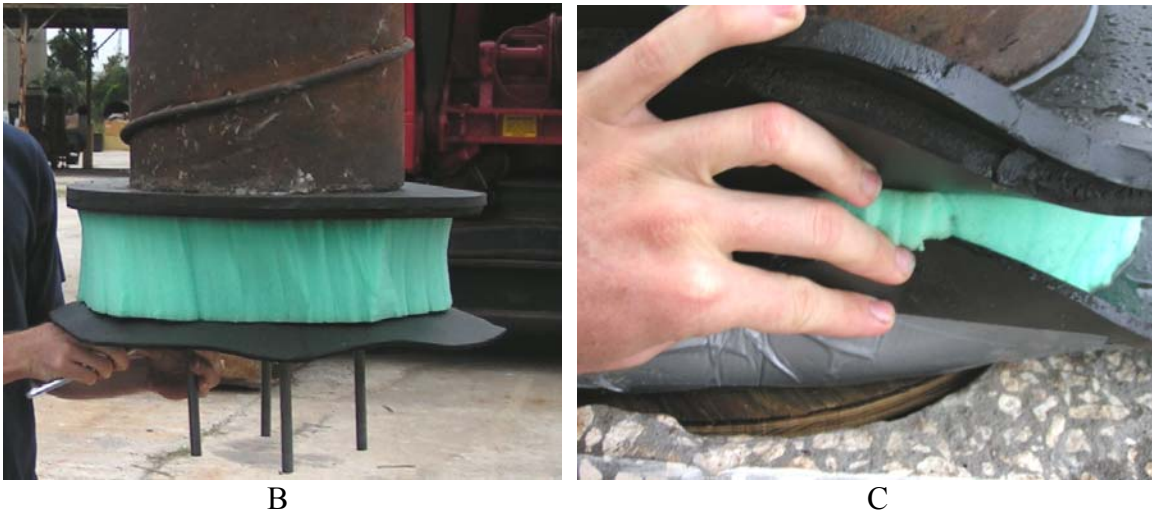
Figure 4-6 Details of the grout plug. A) The dimensions of the grout plug, B) the grout plug is bolted on and compressed with a plywood disc, C) plug in the pile void.
