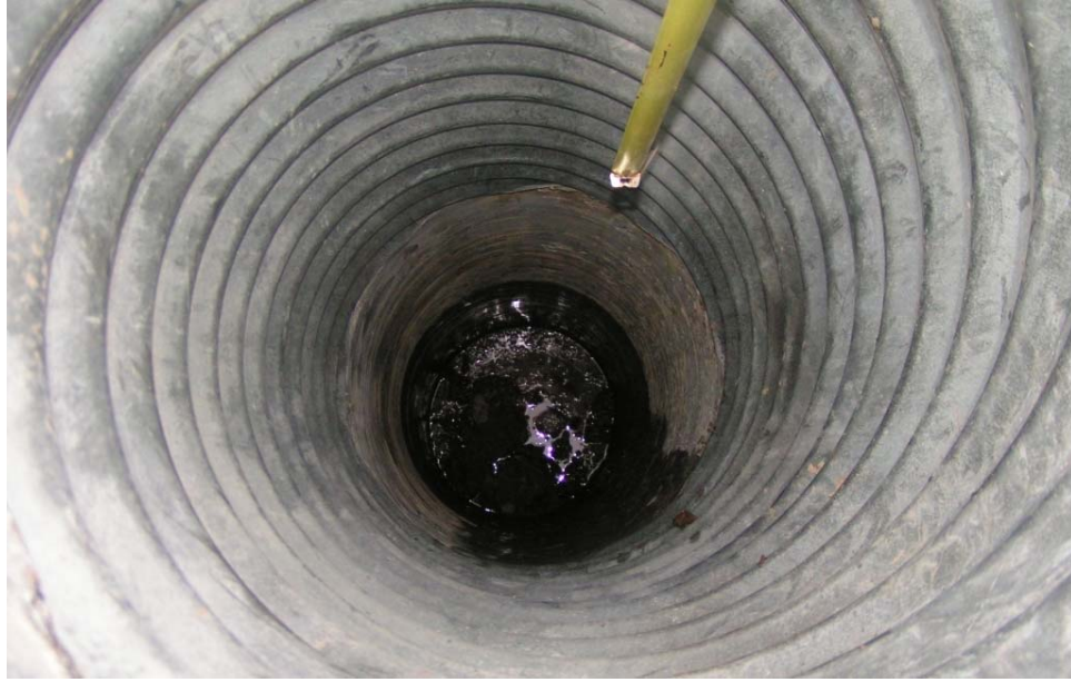
Figure 4-4 Void in each pile after removing cardboard sonotube below 54 inches.
