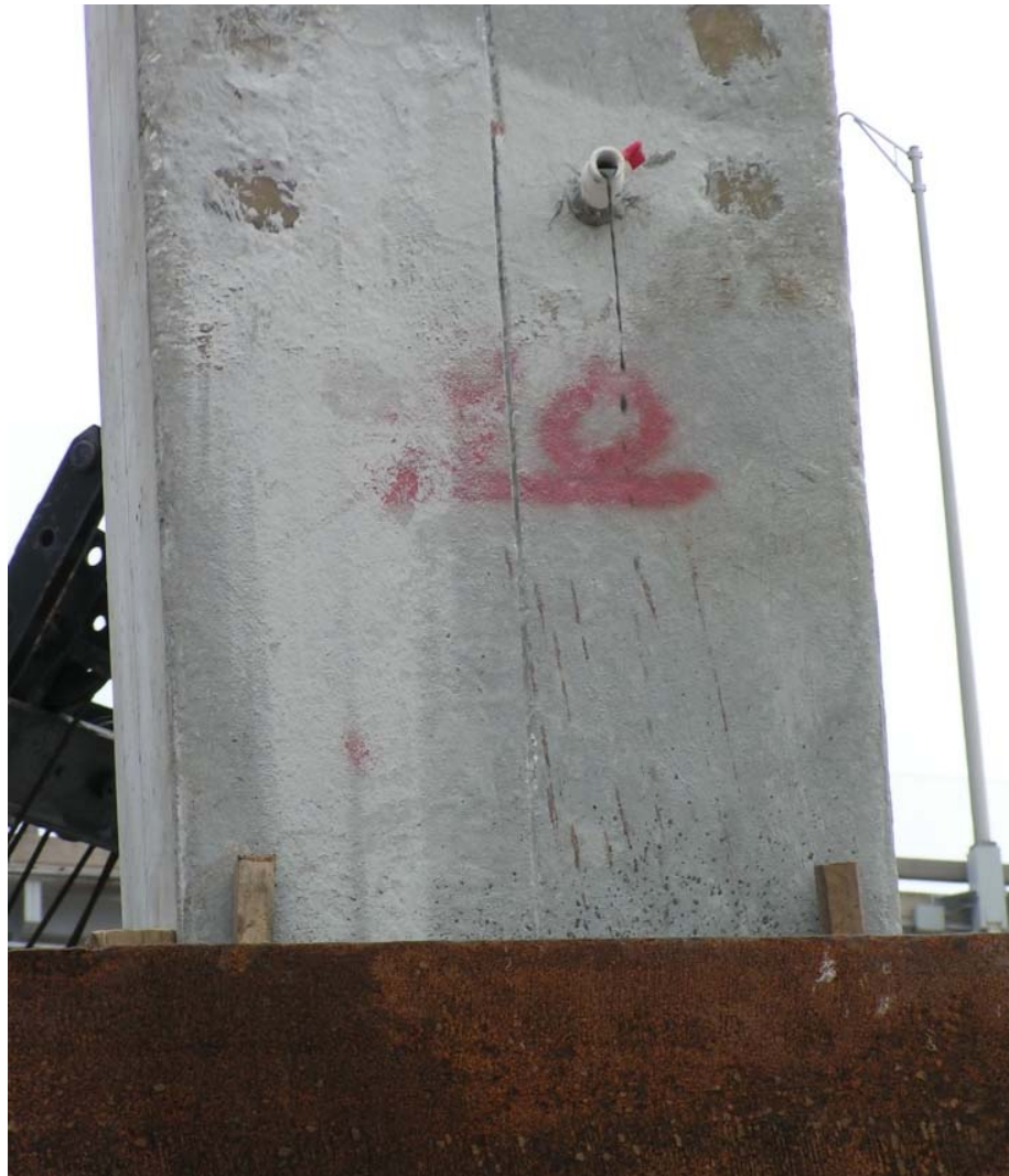
Figure 4-8 Vent hole active and wooden wedges bracing the spliced pile section.
