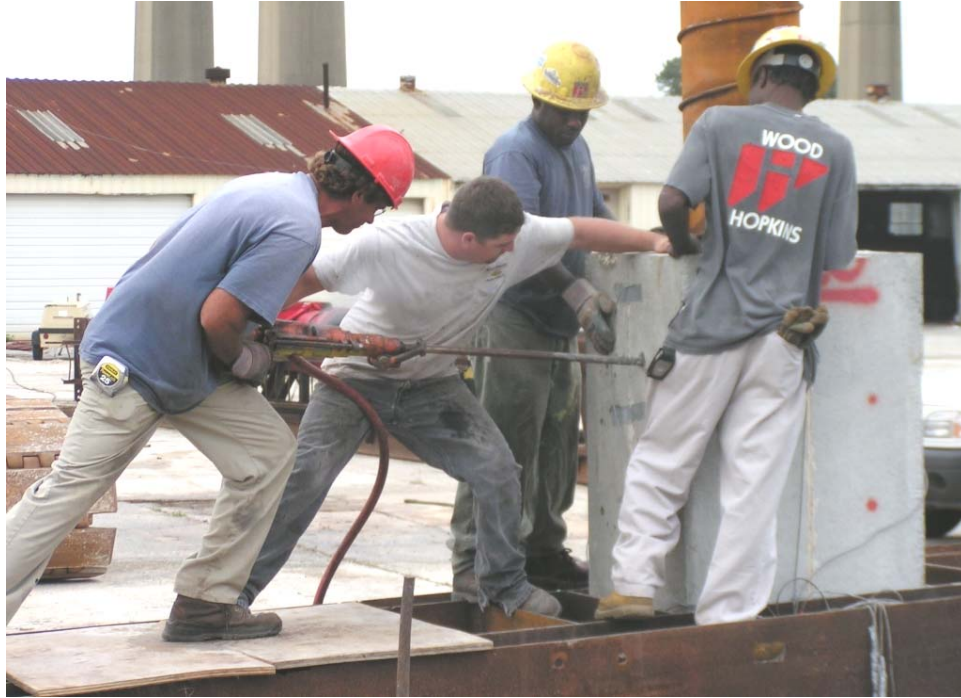
Figure 4-5 Holes drilled to receive bolts to support the steel pipe.
