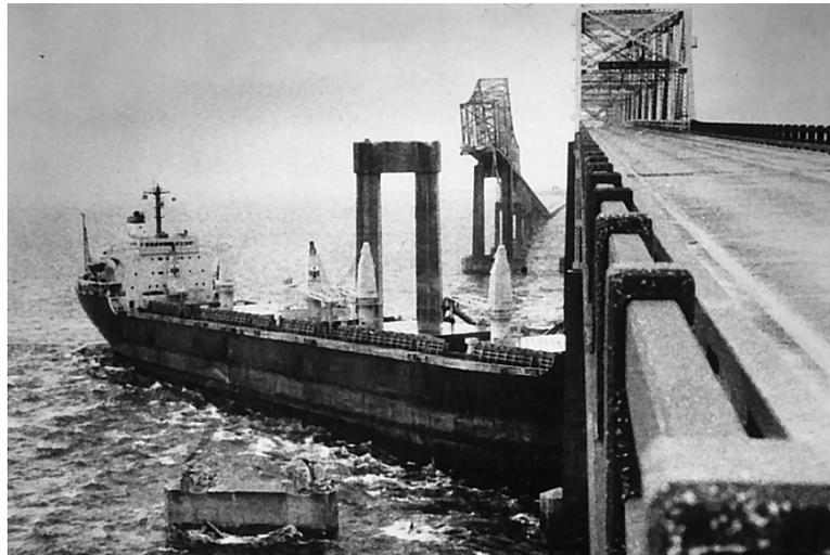
Figure 2.1 Collapse of the Sunshine Skyway Bridge in Florida (1980)
