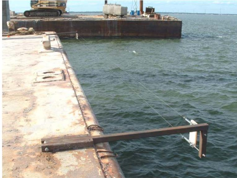
Figure 6.8 Retractable extension arms and tripwires mounted to barge bow
