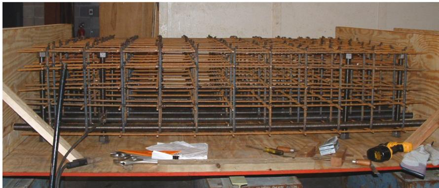
Figure 6.23 Internal steel reinforcing used in impact blocks
