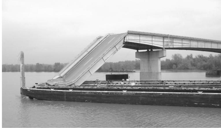
Figure 2.4 Collapse of an Interstate I-40 bridge in Oklahoma (2002)
