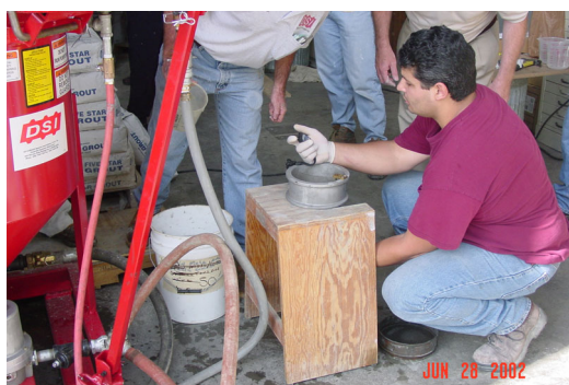
Figure 2 - Flow was checked after mixing and before injection for each grout.
