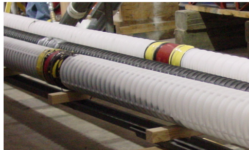
Figure 24 –Grout front in corrugated duct during injection.
