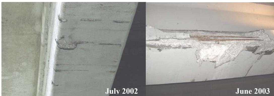
**Figure 15: Vehicle impact damage after strengthening with FRP**
