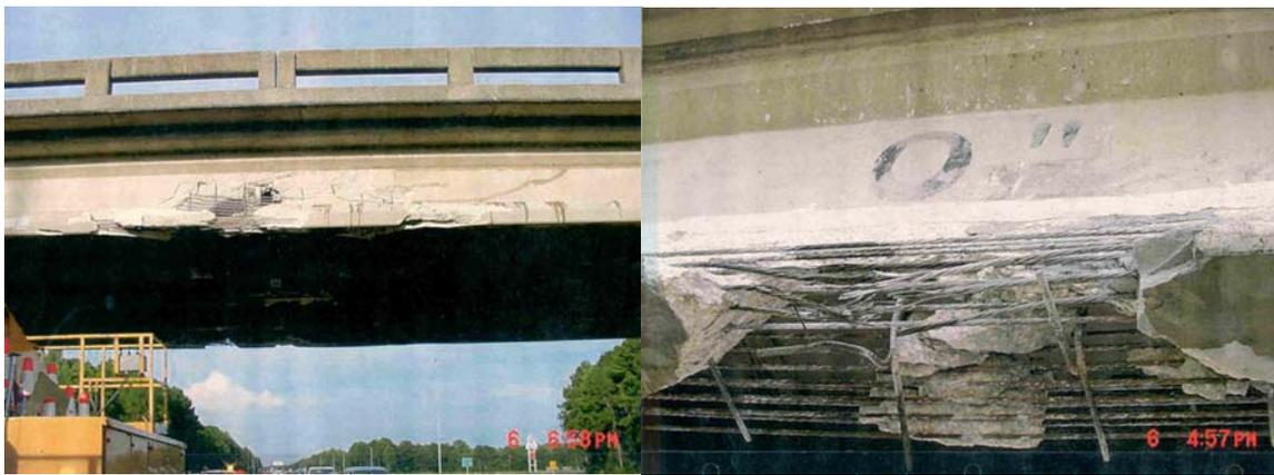
**Figure 14: Original vehicle impact damage that prompted strengthening with FRP**
