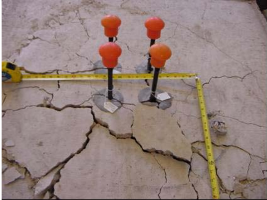
Figure E-9 Typical surface view of cone failure of quadruple fastener anchor group with anchor spacing of 5 inches
