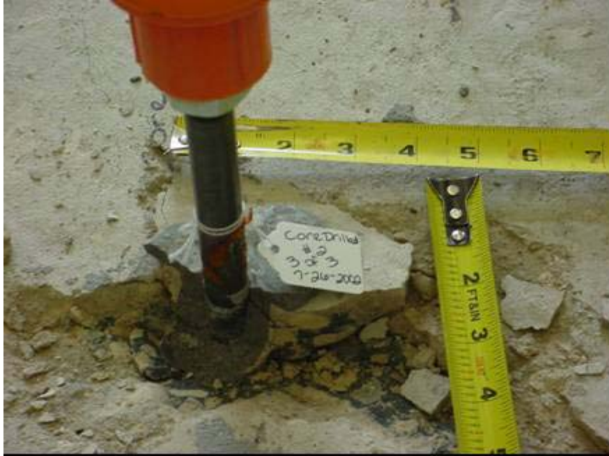
Figure E-3 Grout/concrete bond failure of single core-drilled anchor with secondary shallow cone removed and grout plug exposed
