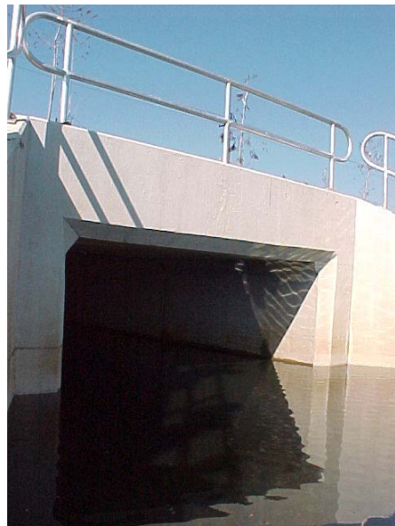
Figure 3.2: Exterior View of Culvert
