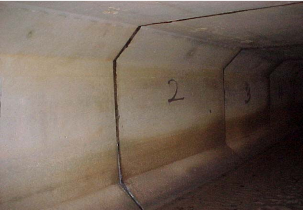
Figure 3.3: Interior View of Culvert Sections
