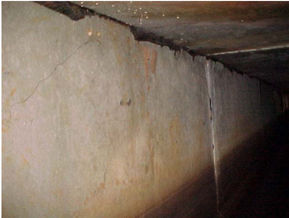
Figure 3.6: Interior View of Culvert
