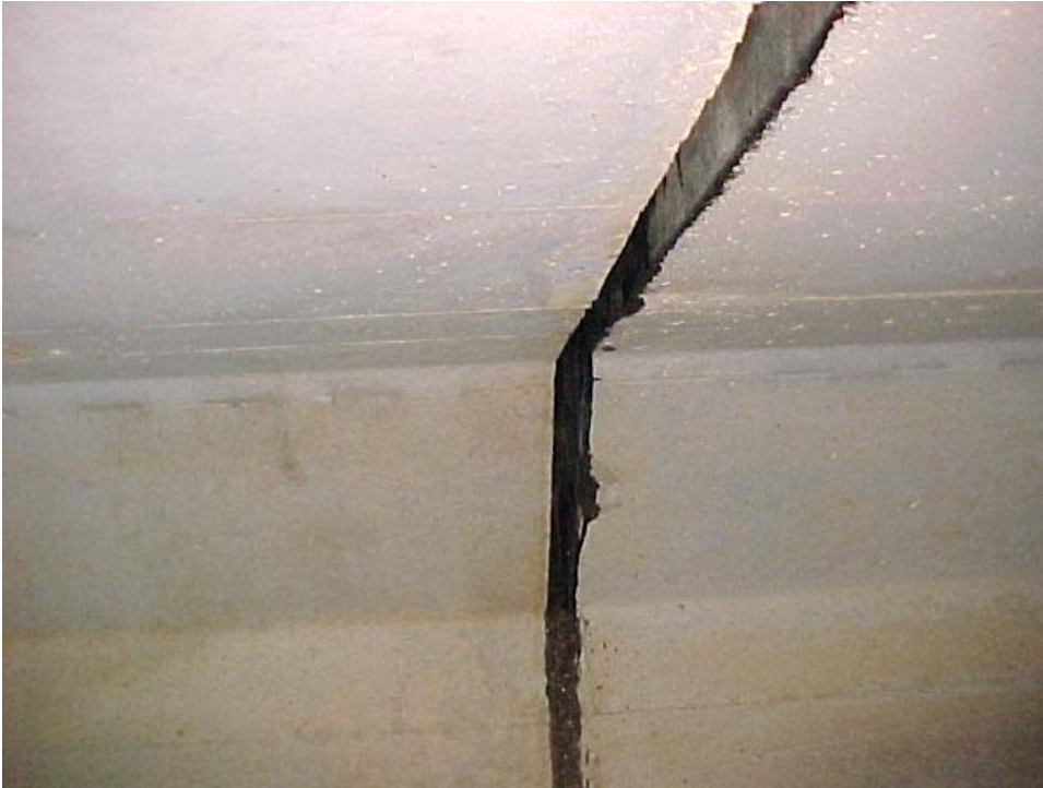
Figure 3.4: Joint Between Culvert Sections
