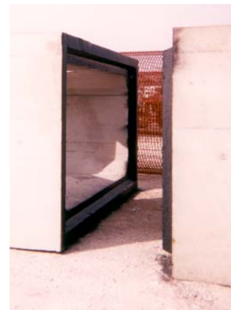
Figure 3.12: Tongue and Groove Joint
