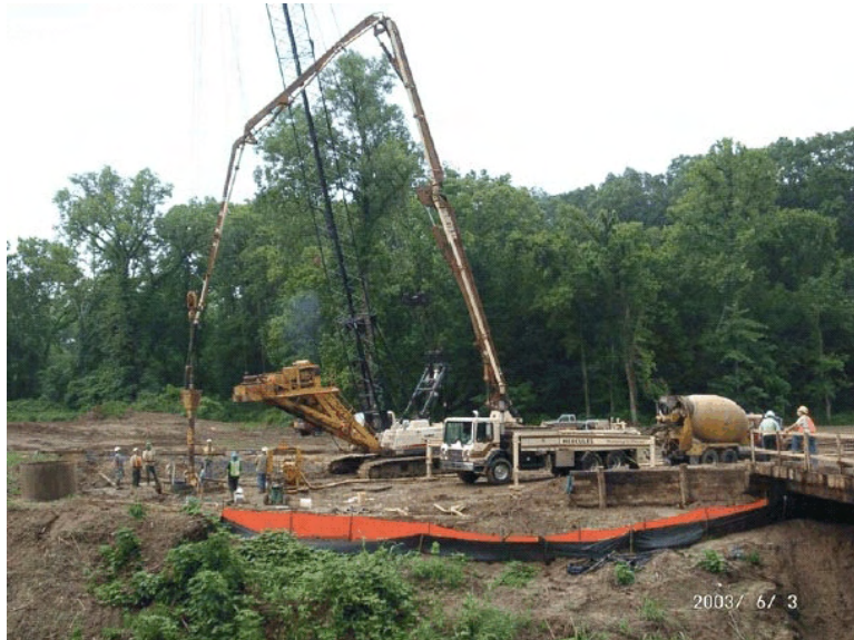
Figure 4-118 Natchez: Concrete placement with a pump truck.
