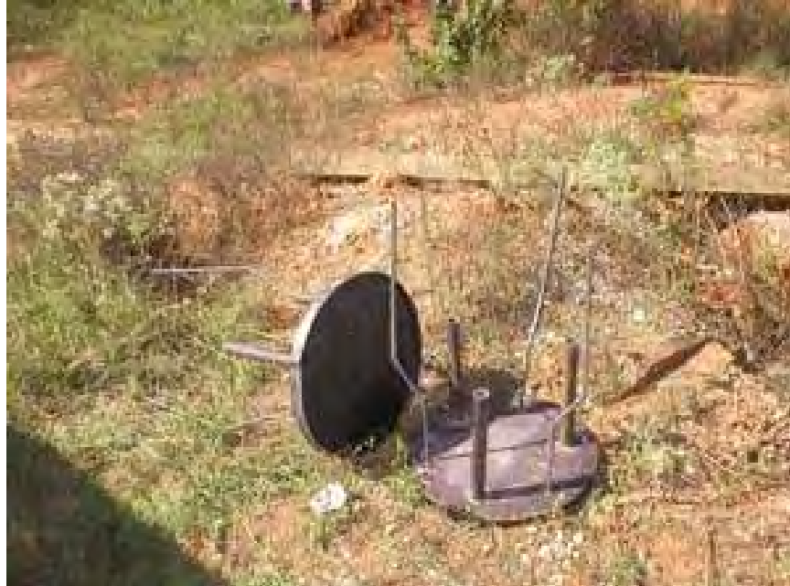
Figure 4-47 NGES Auburn: 24" diameter grout plates.
