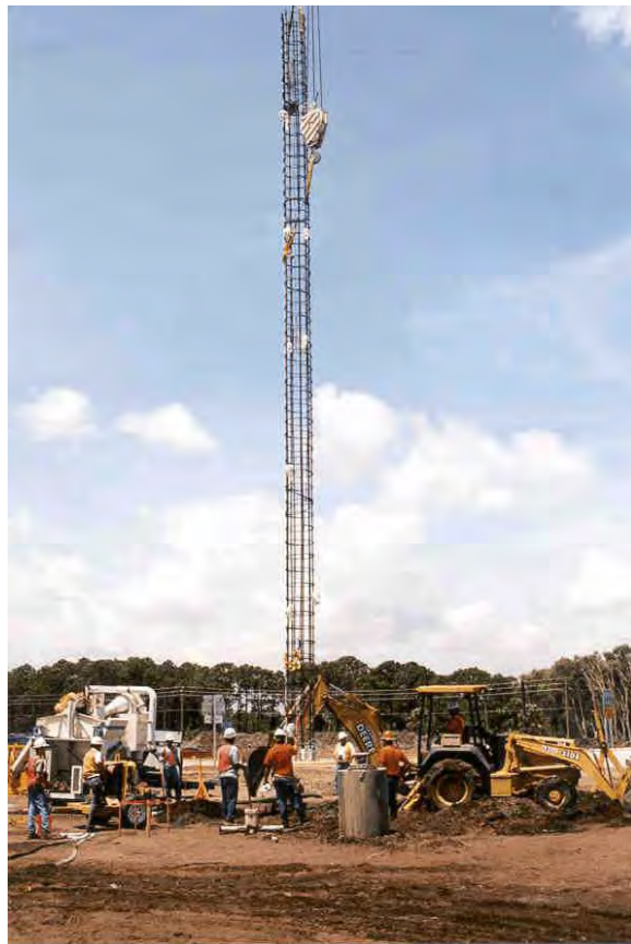
Figure 4-8 PGA Blvd: Reinforcement cage placement.
