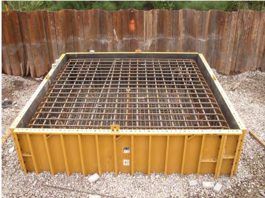
Figure 4-28 PGA Blvd: Pier 2 pile cap reinforcement.
