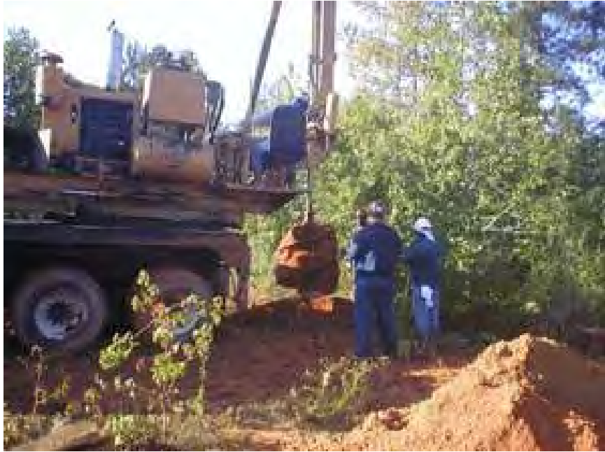
Figure 4-49 NGES Auburn: Drilling of 42" diameter test shafts.
