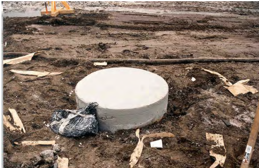
Figure 4-10 PGA Blvd: Control test shaft.
