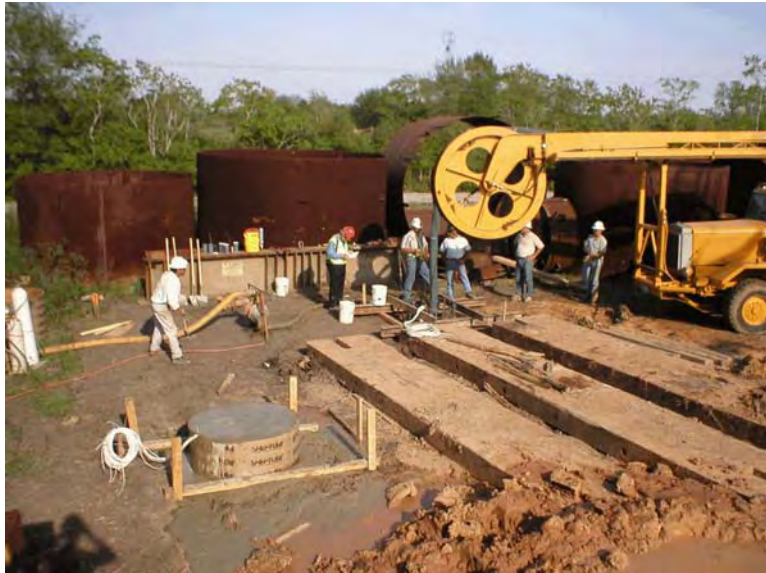
Figure 4-91 TexDOT Demo: Concrete pour.
