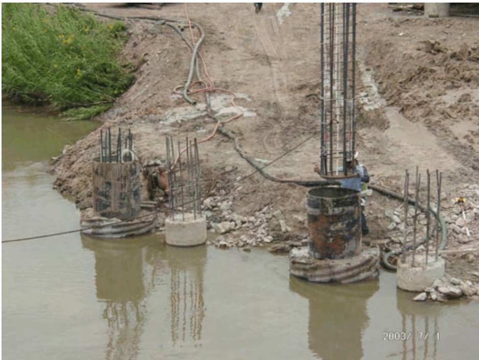
Figure 4-149 FM 507: East shaft cage placement.
