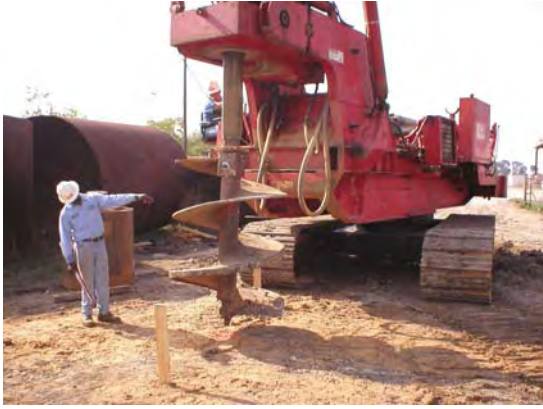
Figure 4-89 TexDOT Demo: Drilling of 48" diameter test shafts.
