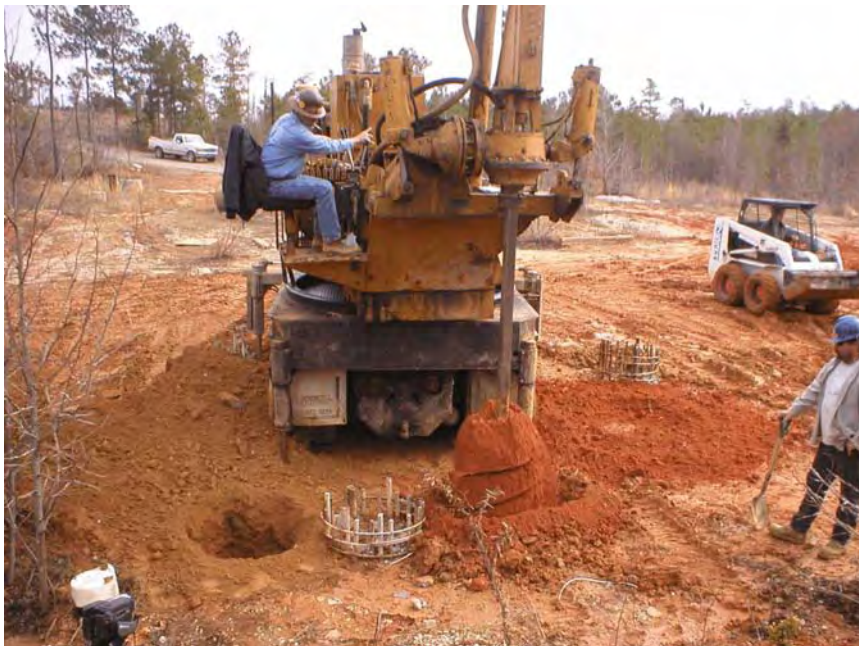
Figure 4-76 NGES Auburn: Exhuming of test shafts.
