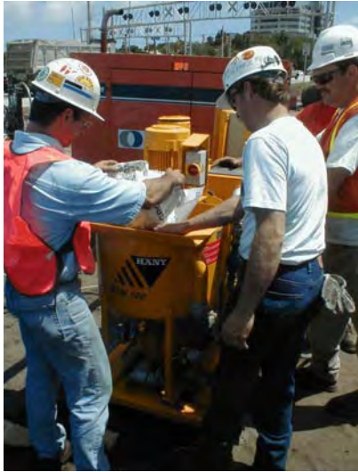
Figure 4-14 PGA Blvd: Post grouting using neat cement with w/c ratio of 0.50.
