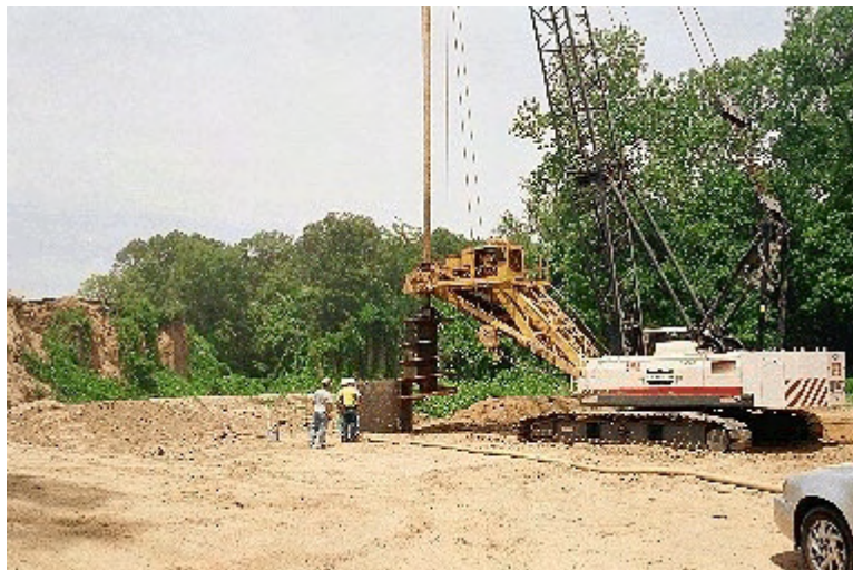
Figure 4-112 Natchez: Drilling of test shaft with isolation casing.
