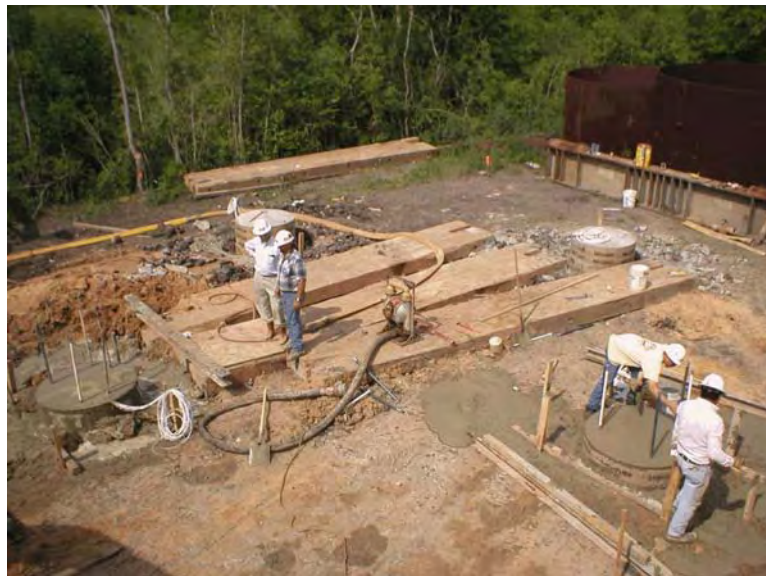
Figure 4-92 TexDOT Demo: Test site.
