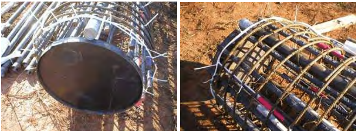
Figure 4-48 NGES: Grout plate, lower strain gages, and CSL tubes installation.
