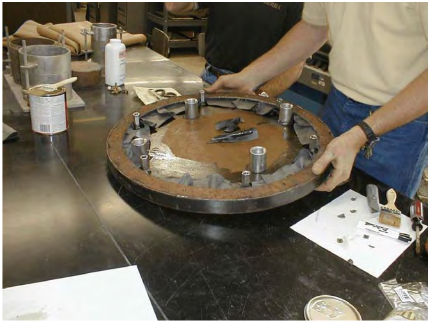
Figure 4-4 PGA Blvd: Installation of scuff ring on grout plate.
