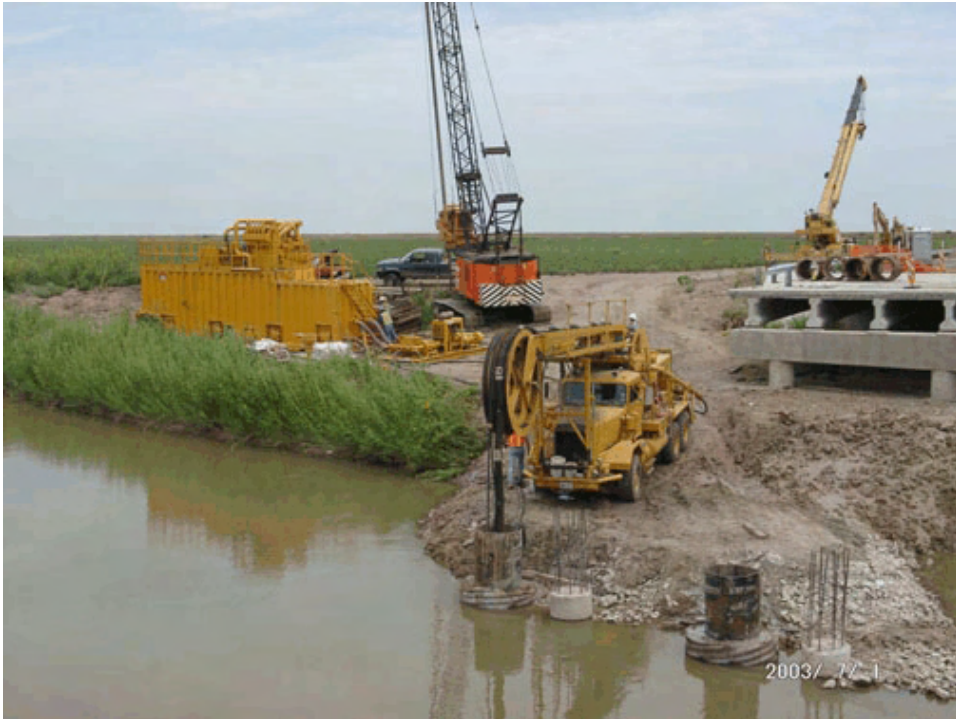
Figure 4-144 FM 507: De-sanding of the west shaft.
