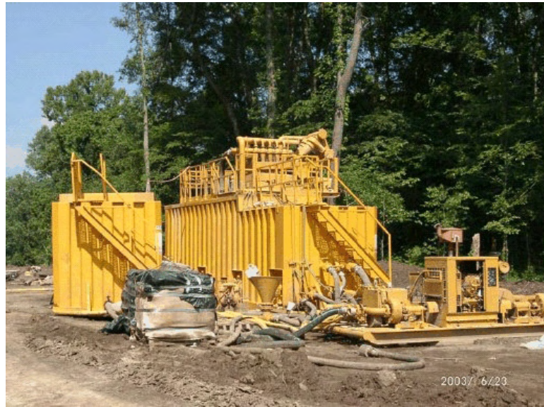
Figure 4-113 Natchez: Slurry tank and de-sanding unit.
