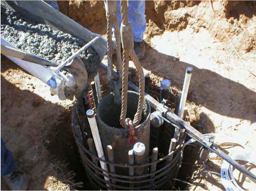
Figure 4-52 NGES Auburn: Drilled shaft concrete pour.
