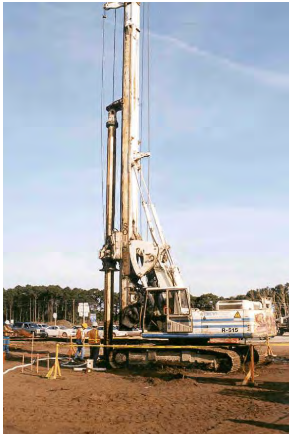
Figure 4-6 PGA Blvd: Drilling of test shafts.
