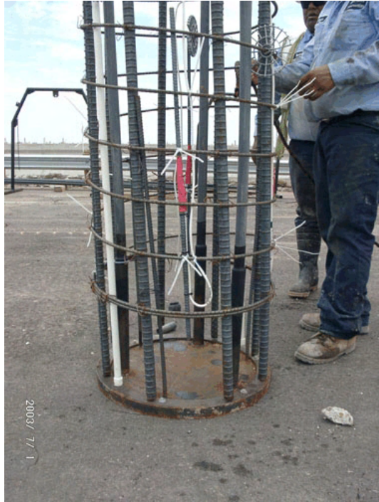
Figure 4-148 FM 507: Grout plate attached to reinforcement cage prior to placement.
