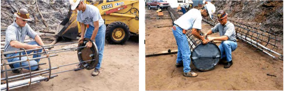
Figure 4-5 PGA Blvd: Installation of grout plate.
