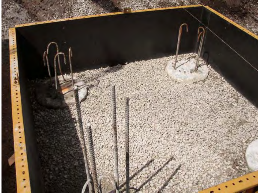
Figure 4-27 PGA Blvd: Pier 2 pile cap formation.
