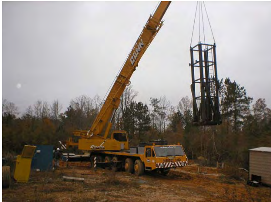
Figure 4-67 NGES Auburn: Statnamic test setup.
