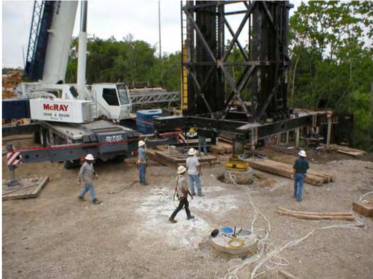
Figure 4-103 TexDOT Demo: Statnamic setup
