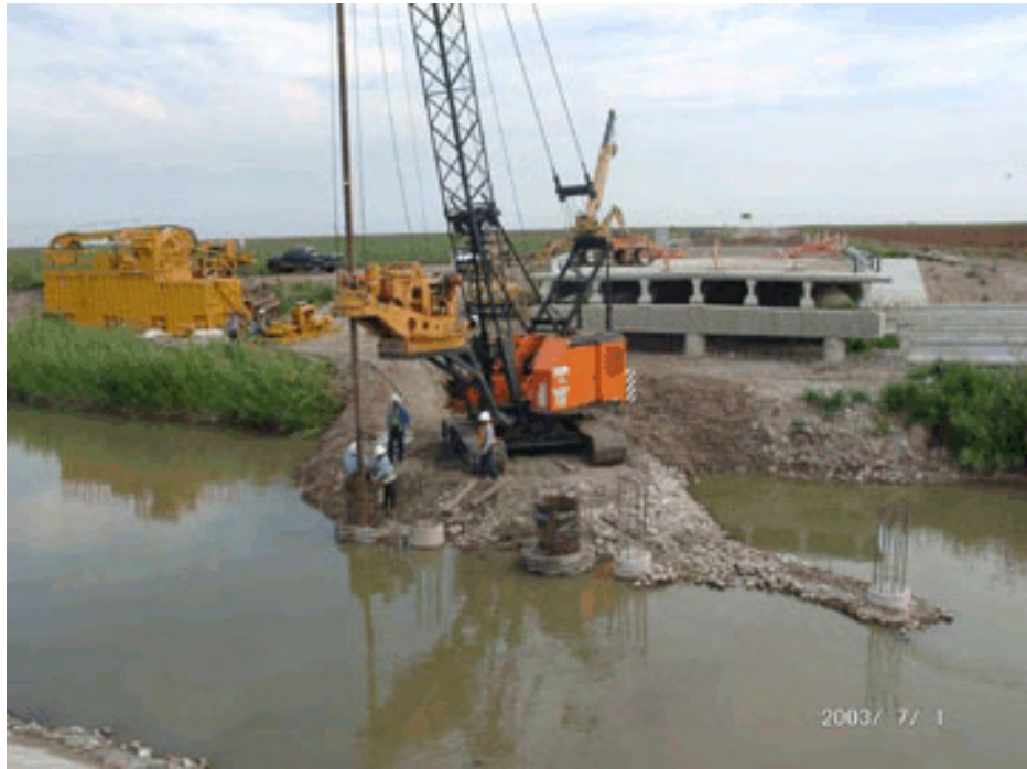
Figure 4-142 FM 507: Setup and drilling of the west shaft.
