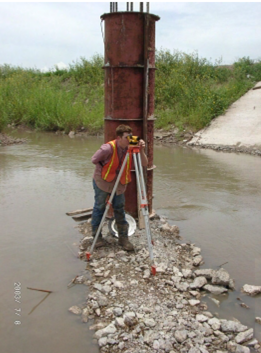
Figure 4-155 FM 507: Field surveying during grouting.
