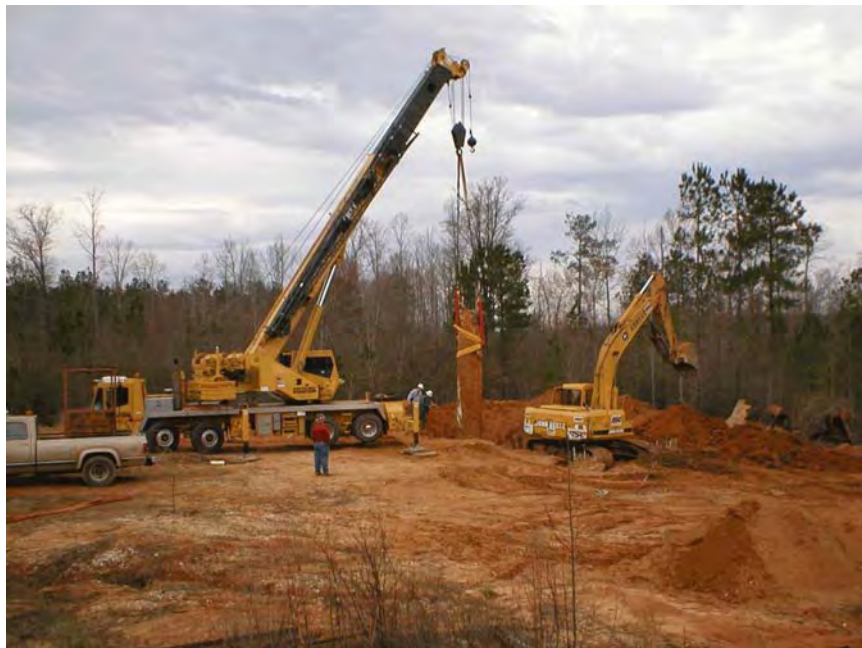
Figure 4-78 NGES Auburn: Shaft extraction.
