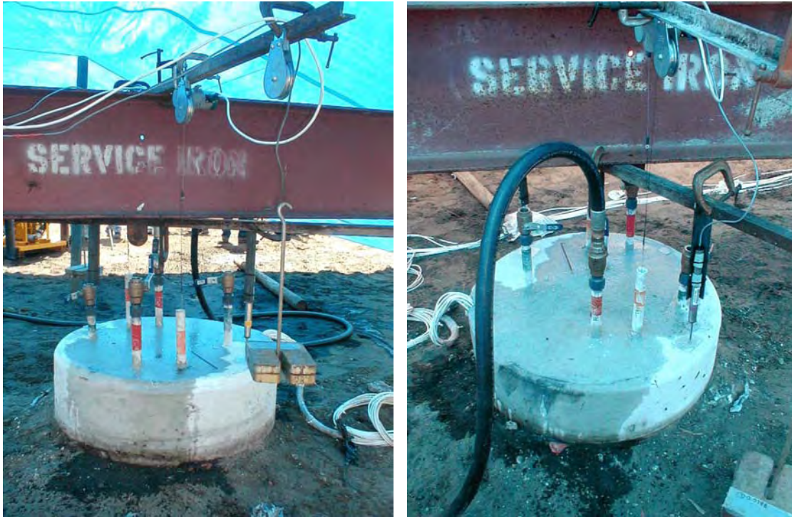
Figure 4-11 PGA Blvd: Post grout instrumentation setup.
