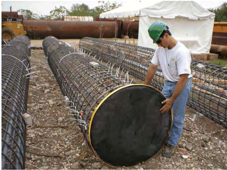
Figure 4-87 TexDOT Demo: Grout plate installation.
