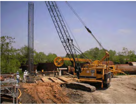
Figure 4-90 TexDOT Demo: Reinforcement cage placement.
