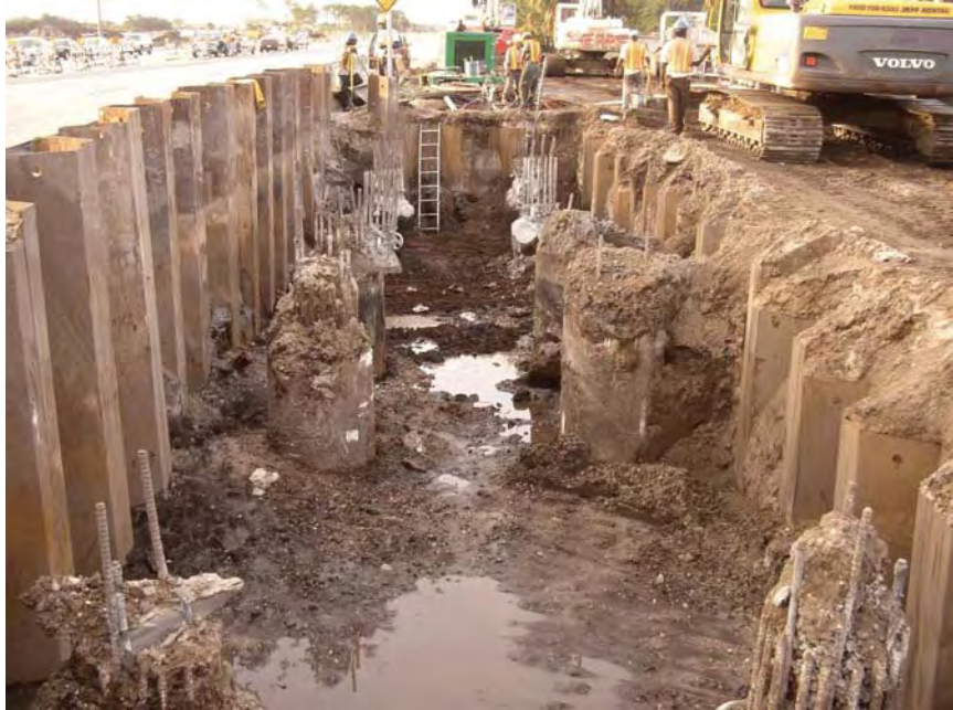
Figure 4-25 PGA Blvd: Pier 3 shafts prior to post grouting.
