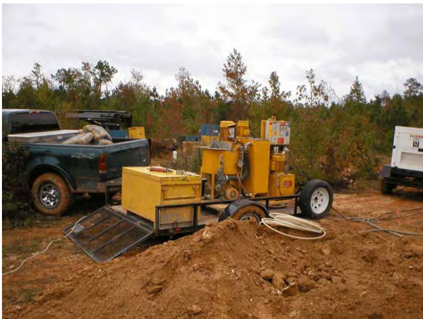
Figure 4-56 NGES Auburn: Grout pump.
