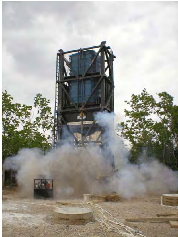
Figure 4-104 TexDOT Demo: Statnamic load test
