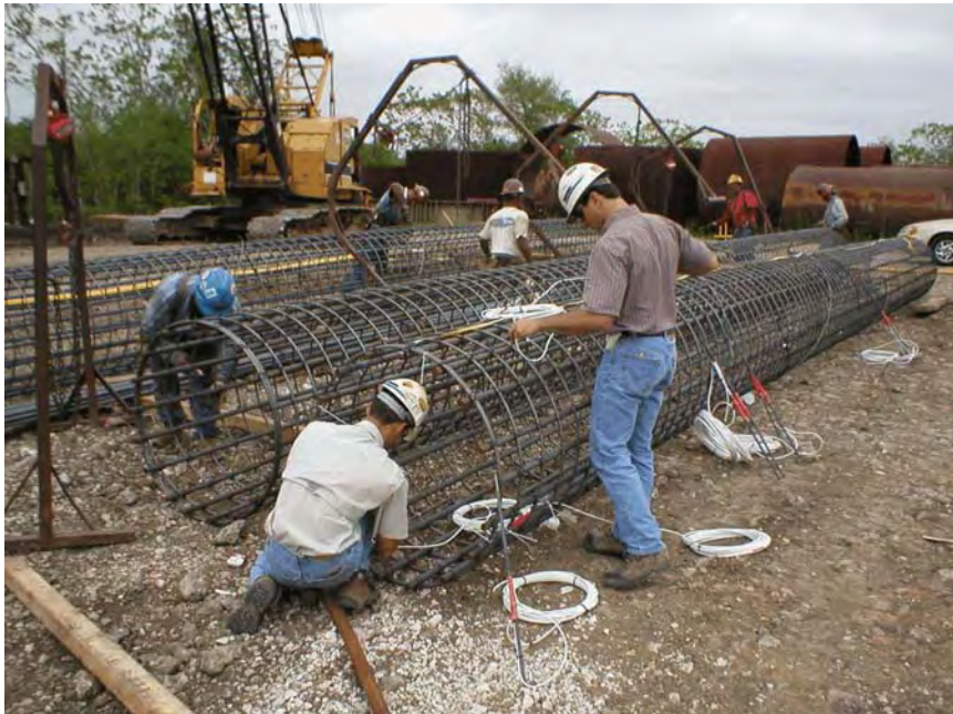
Figure 4-85 TexDOT Demo: Strain gage installation.
