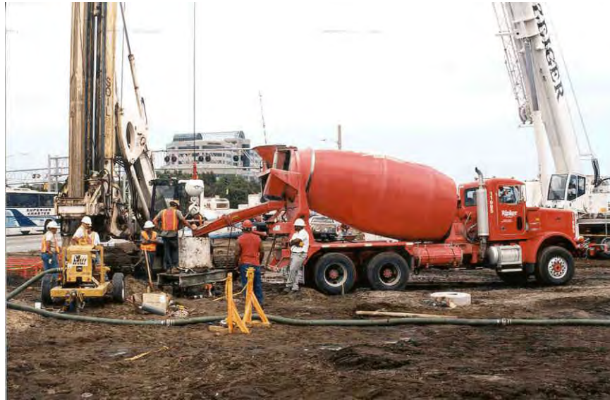
Figure 4-9 PGA Blvd: Concrete pour of test shafts.
