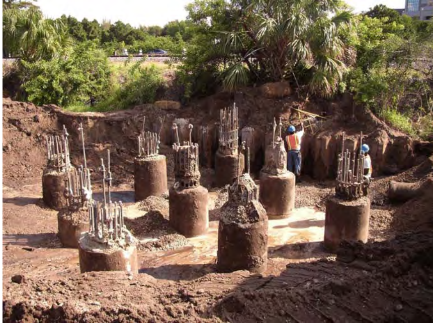
Figure 4-31 PGA Blvd: Southwest ramp Pier 2 production shafts.
