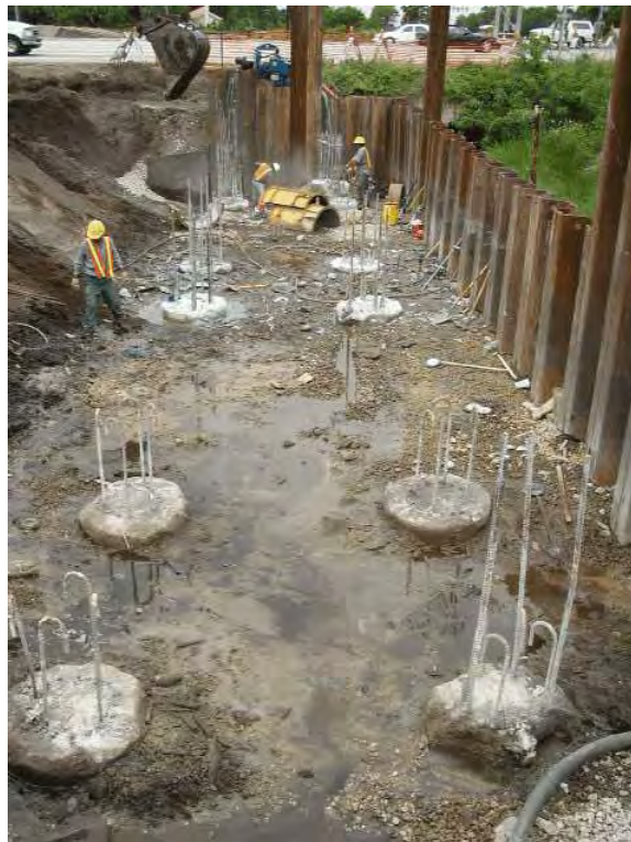
Figure 4-26 PGA Blvd: Pier 2 prior to post grouting.
