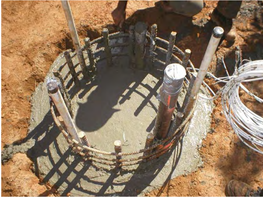
Figure 4-53 NGES Auburn: Top of shaft finishing.
