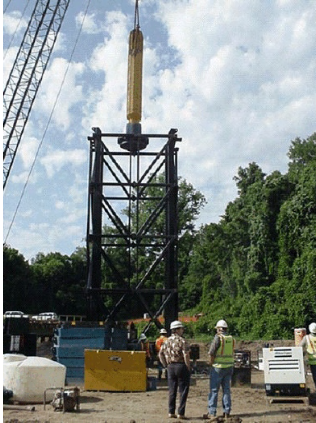
Figure 4-129 Natchez: Statnamic load test setup.
