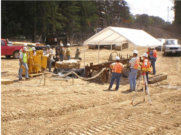
Figure 4-121 Natchez: Post grout setup and testing.
