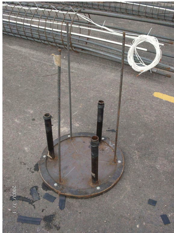
Figure 4-147 FM 507: 24" grout plate.
