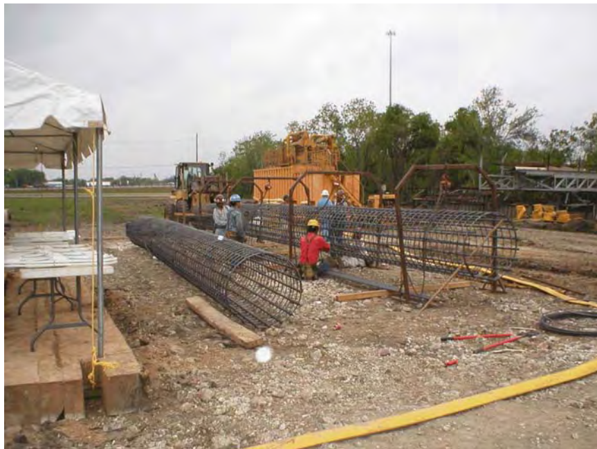
Figure 4-84 TexDOT Demo: Reinforcement cage construction.
