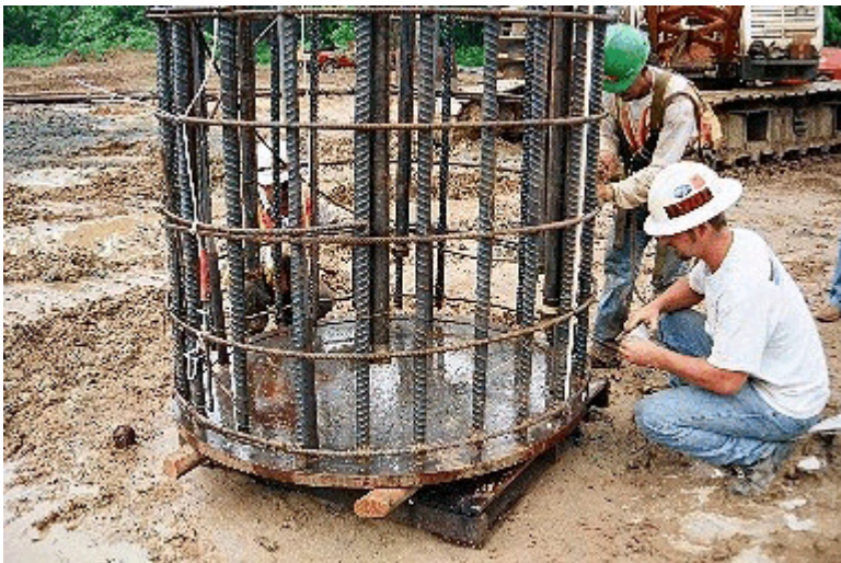
Figure 4-116 Natchez: Grout plate installation.
