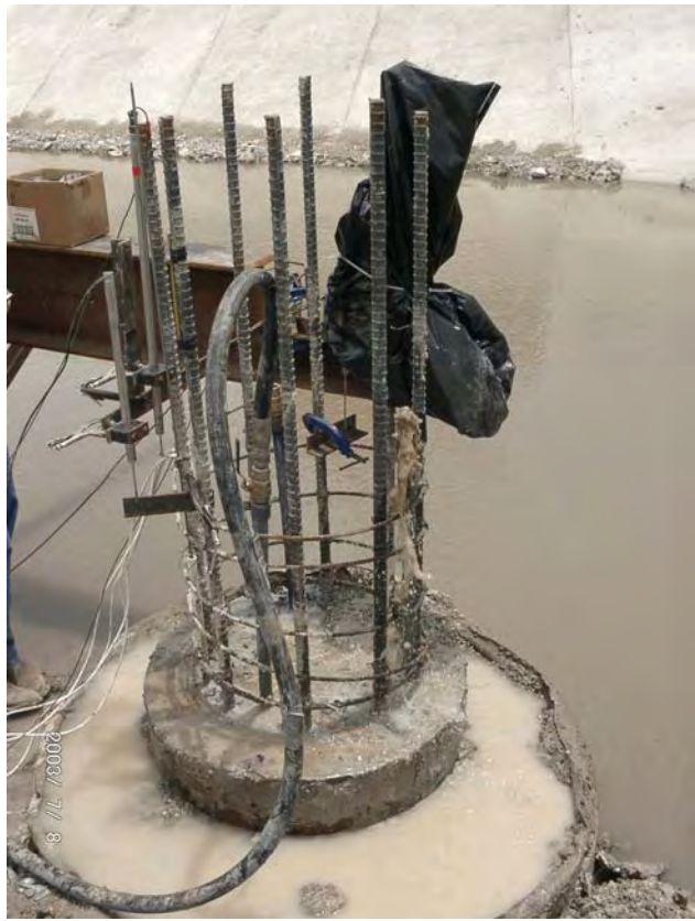
Figure 4-153 FM 507: Grouting of the west shaft.
