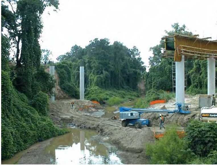
Figure 4-137 Natchez: Production bridge bents.
