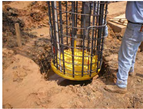
Figure 4-90 TexDOT Demo: Reinforcement cage placement.
