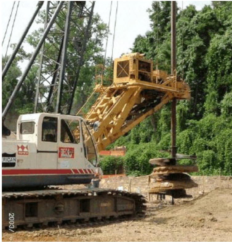
Figure 4-111 Natchez: Crane mounted drill rig.
