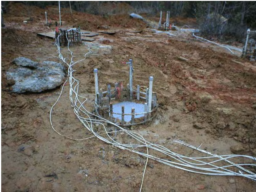
Figure 4-54 NGES Auburn: Test shafts.
