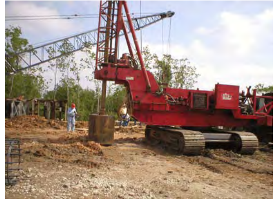
Figure 4-89 TexDOT Demo: Drilling of 48" diameter test shafts.
