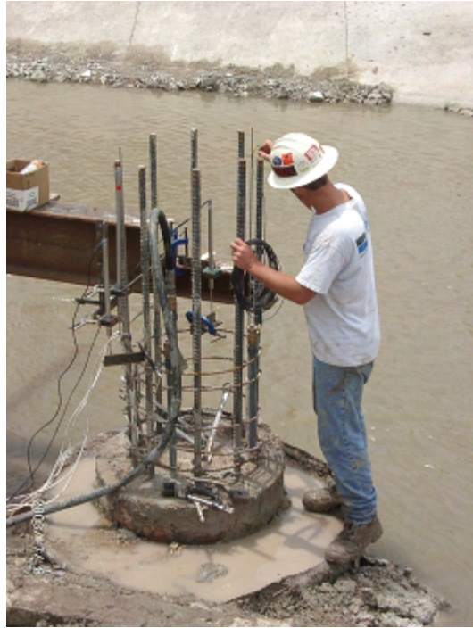
Figure 4-156 FM 507: Instrumentation setup on the west shaft.
