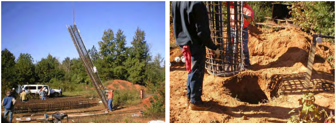
Figure 4-51 NGES Auburn: Reinforcement cage installation.
