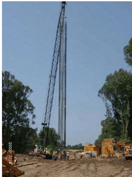
Figure 4-136 Natchez: Bent 8 cage placement.
