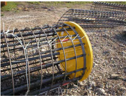
Figure 4-88 TexDOT Demo: Grout plates and strain gages installed.
