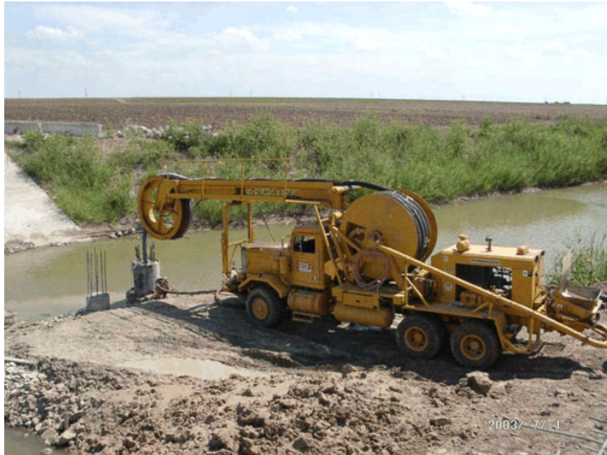
Figure 4-150 FM 507: Concrete placement in west shaft.
