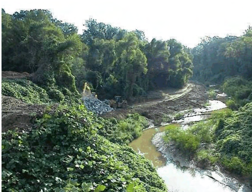
Figure 4-134 Natchez: Production site preparation.
