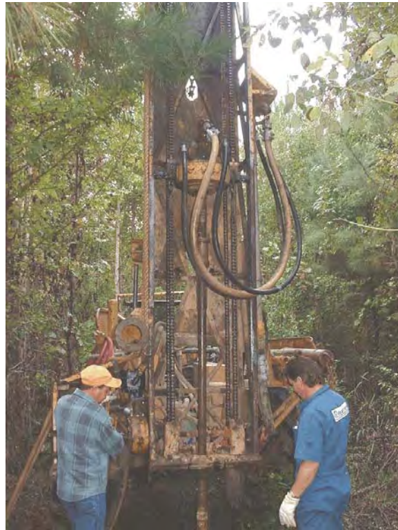
Figure 4-110 Natchez: SPT testing.
