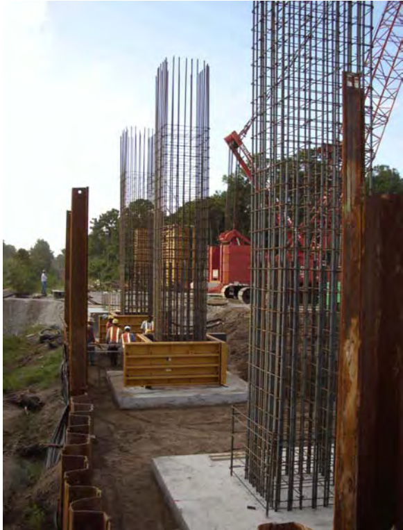
Figure 4-30 PGA Blvd: Pier 2.
