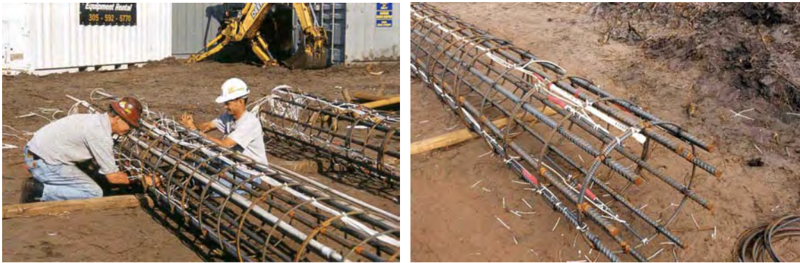
Figure 4-1 PGA Blvd: Installation of strain gages and toe accelerometer.
