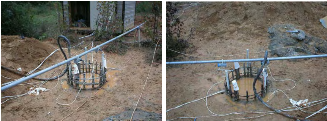
Figure 4-58 NGES Auburn: Post grouting test setup.
