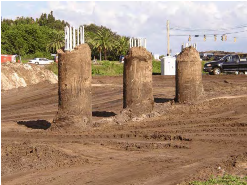
Figure 4-24 PGA Blvd: Post grouted production shafts.
