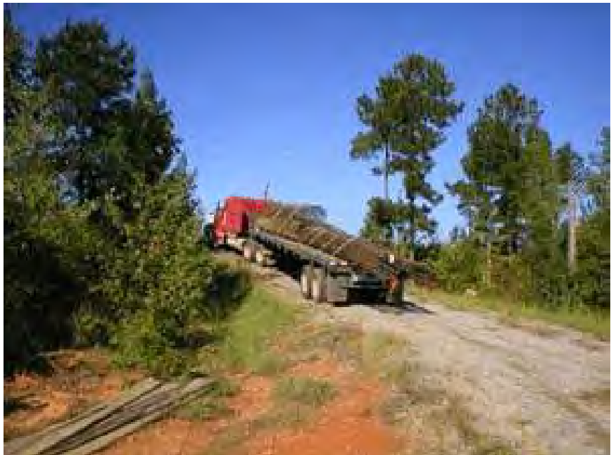
Figure 4-46 NGES Auburn: Reinforcement cages.
