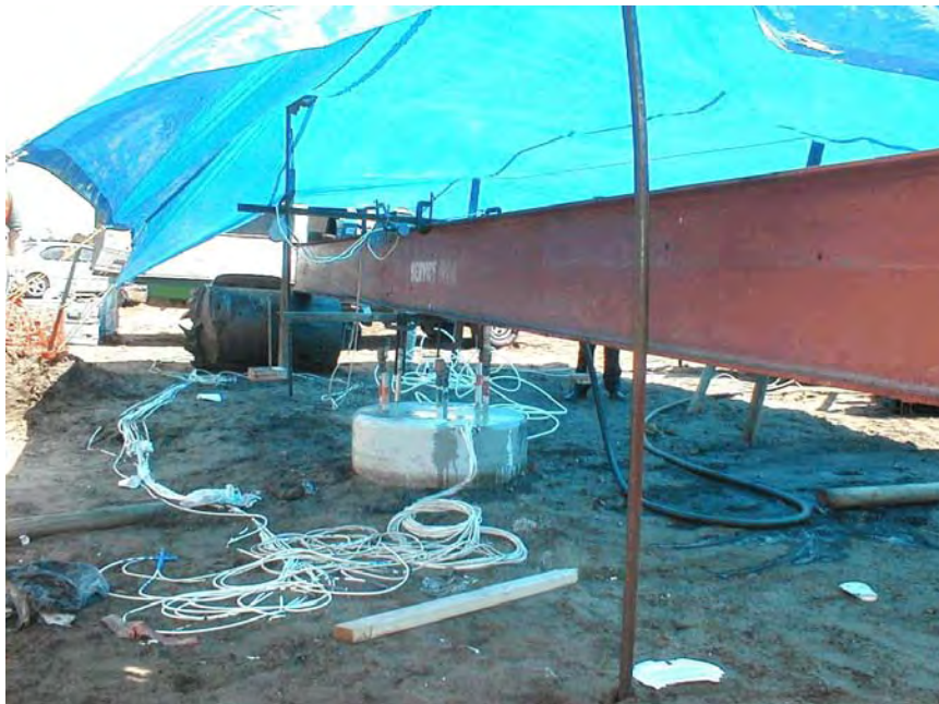
Figure 4-12 PGA Blvd: Post grouting setup.
