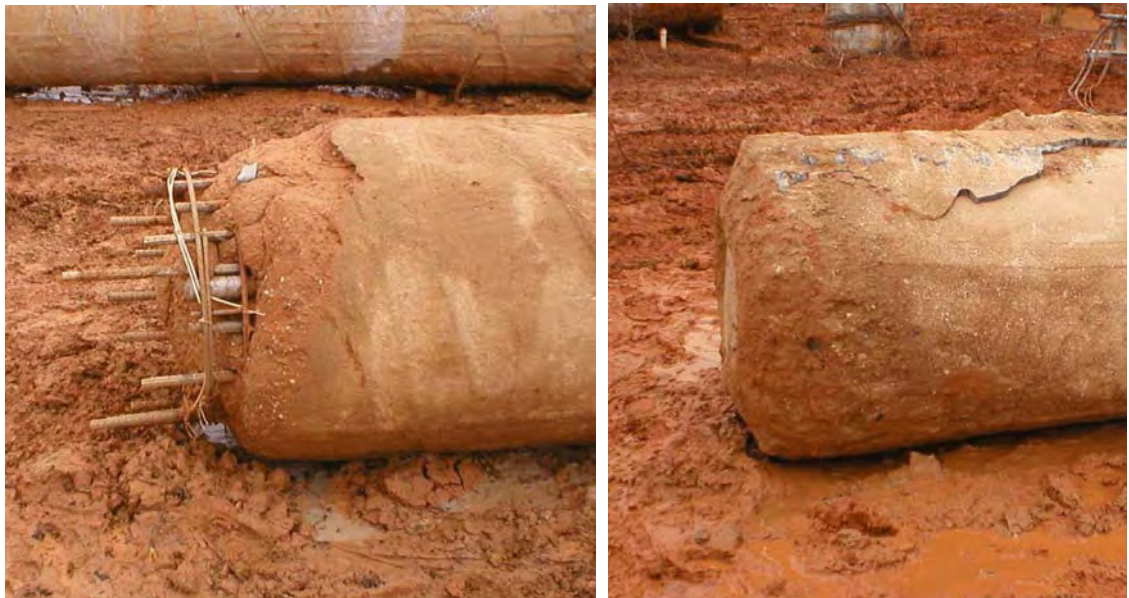
Figure 4-80 NGES Auburn: UngROUTED shaft vs. Grouted shaft.
