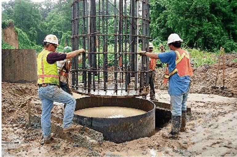
Figure 4-117 Natchez: Reinforcement cage installation.
