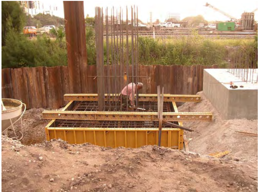
Figure 4-29 PGA Blvd: Pier 2 pile cap reinforcement with column reinforcement.
