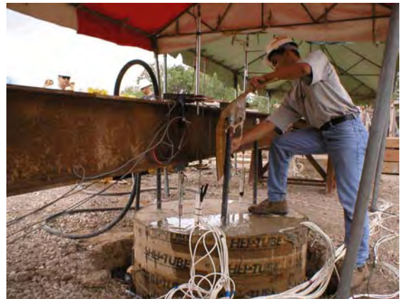
Figure 4-94 TexDOT Demo: Post grout setup and flushing of lines.
