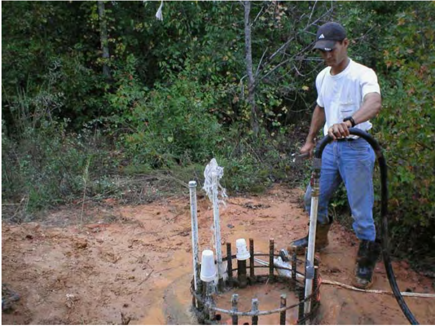
Figure 4-57 NGES Auburn: Flushing grout lines.
