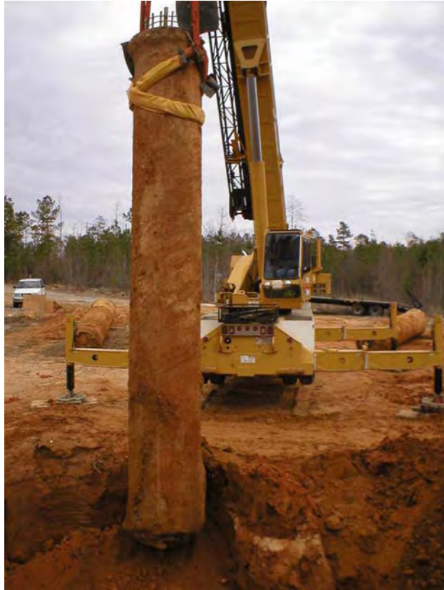
Figure 4-79 NGES Auburn: Grouted shaft extraction.
