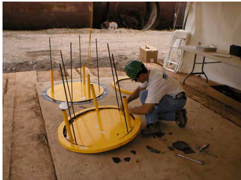
Figure 4-86 TexDOT Demo: Installation of rubber membrane on grout plates.
