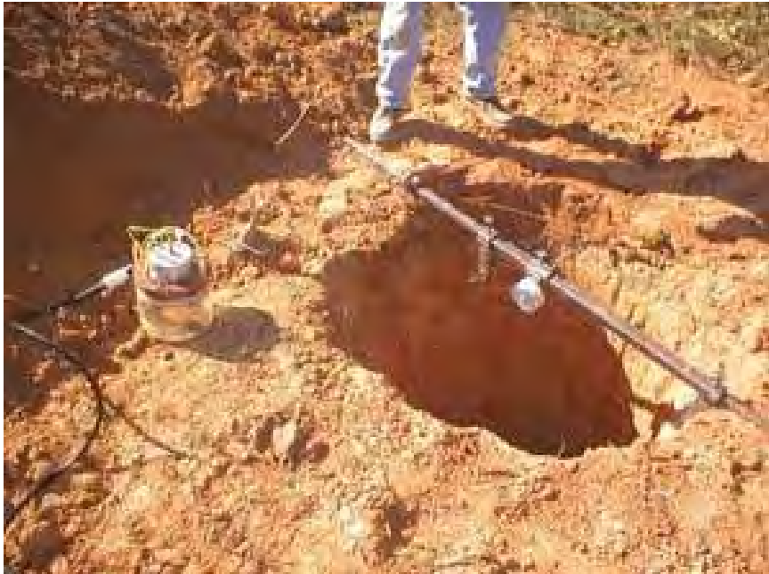
Figure 4-50 NGES Auburn: FDOT Borescope inspection.
