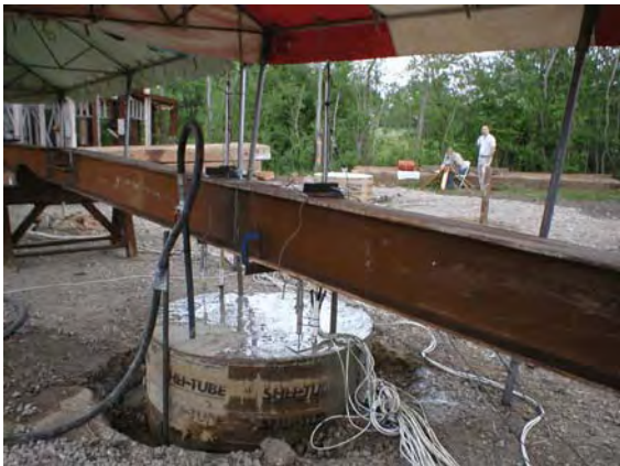
Figure 4-94 TexDOT Demo: Post grout setup and flushing of lines.
