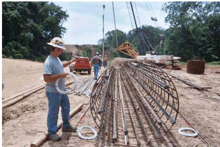
Figure 4-114 Natchez: Strain gage installation.
