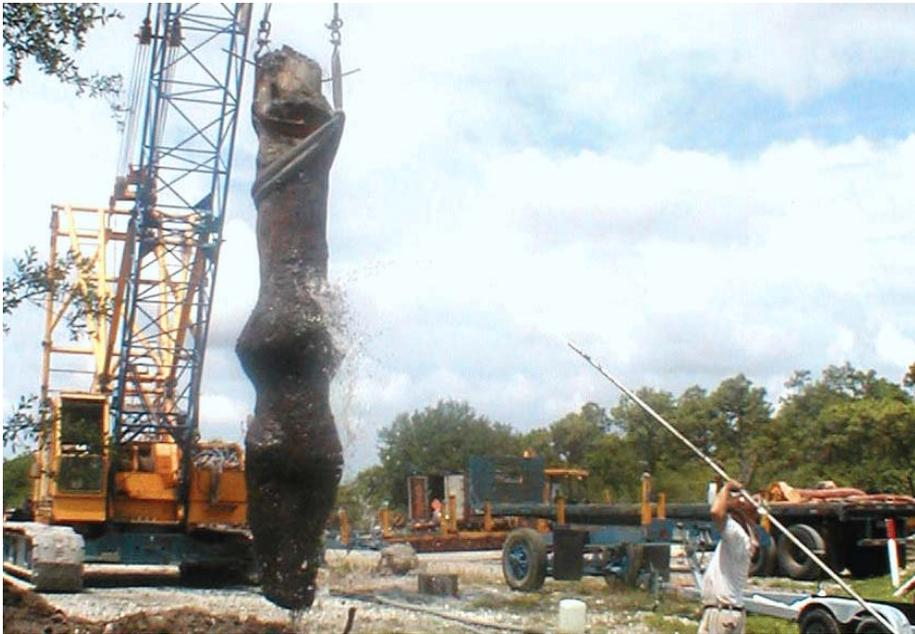
Figure 4-36. Site II exhumed Control Shaft.
