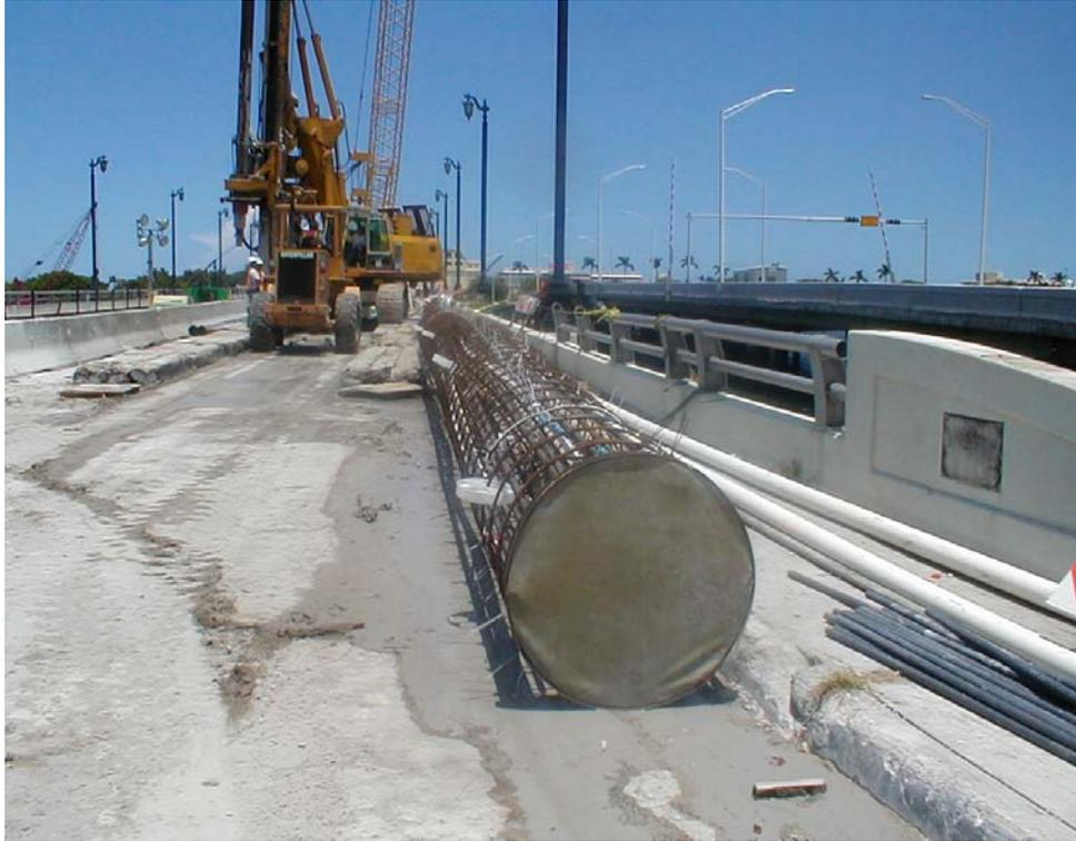
Figure 4-37. Site III LT-2 cage with flat-jack grouting apparatus.
