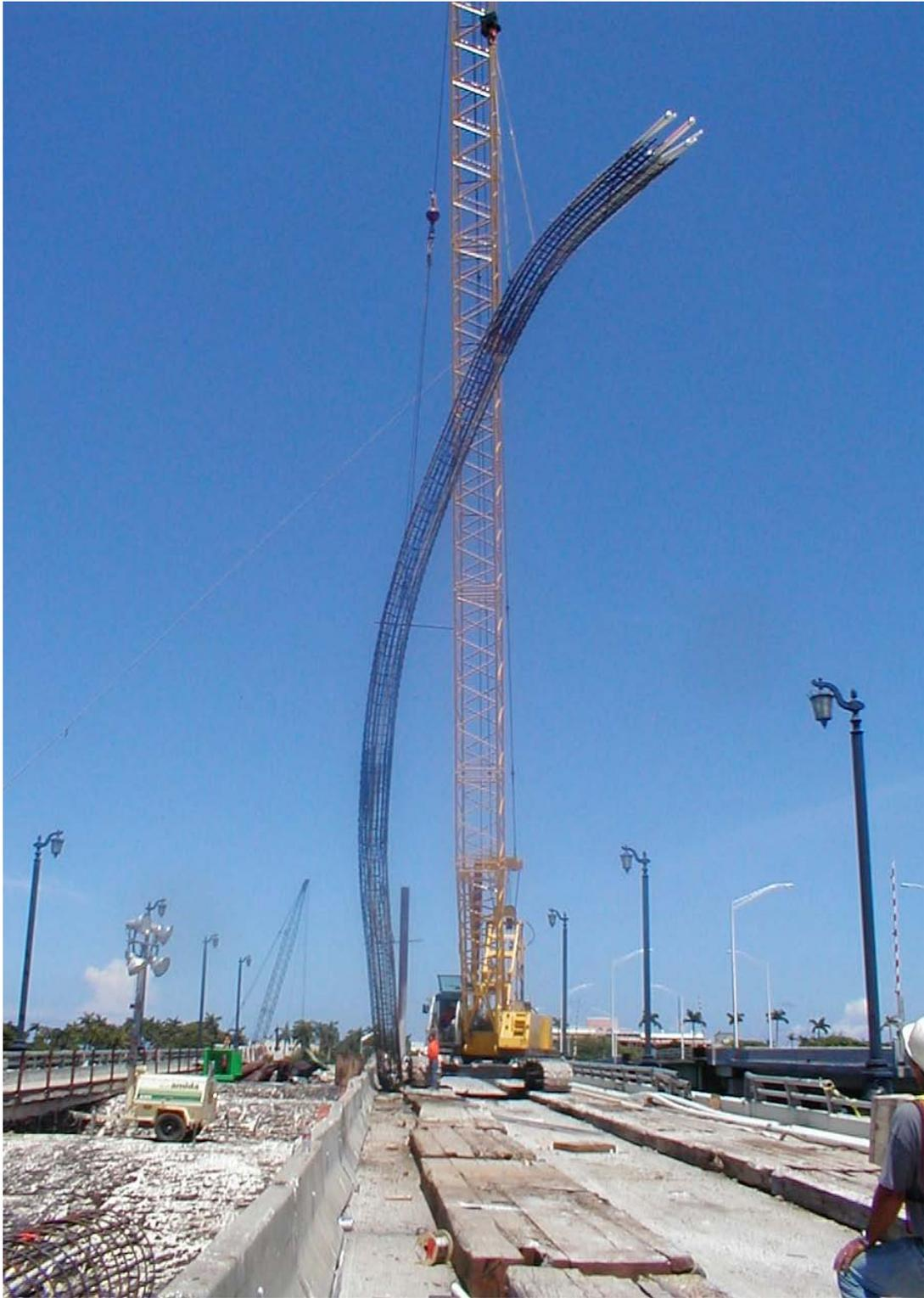
Figure 4-40. Kobelco crane lifting cage for Site III LT-3.
