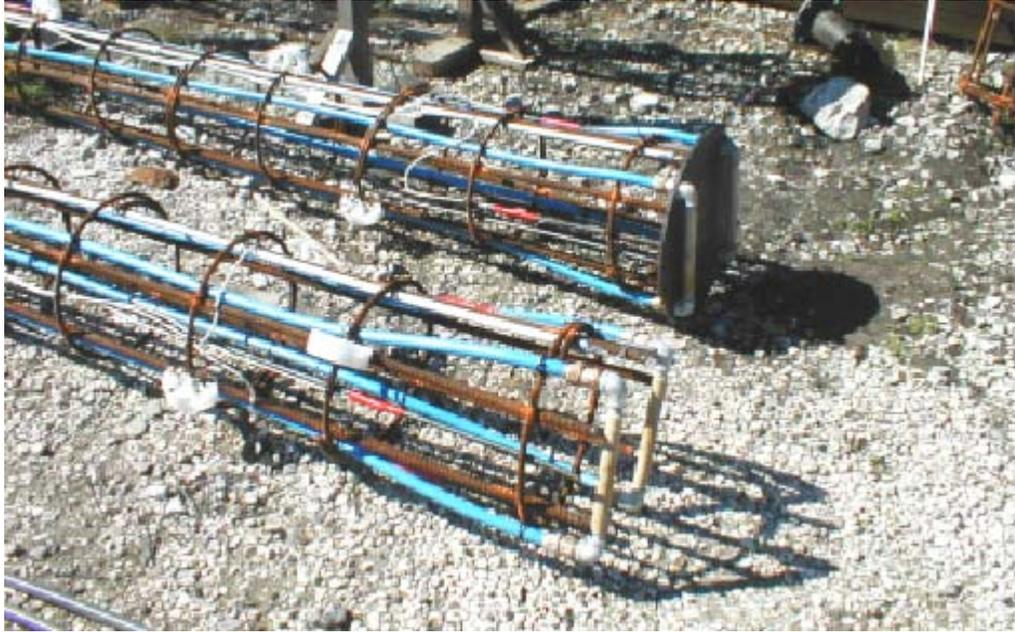
Figure 4-22. Site I sleeve-port apparatus tied into reinforcing cages.
