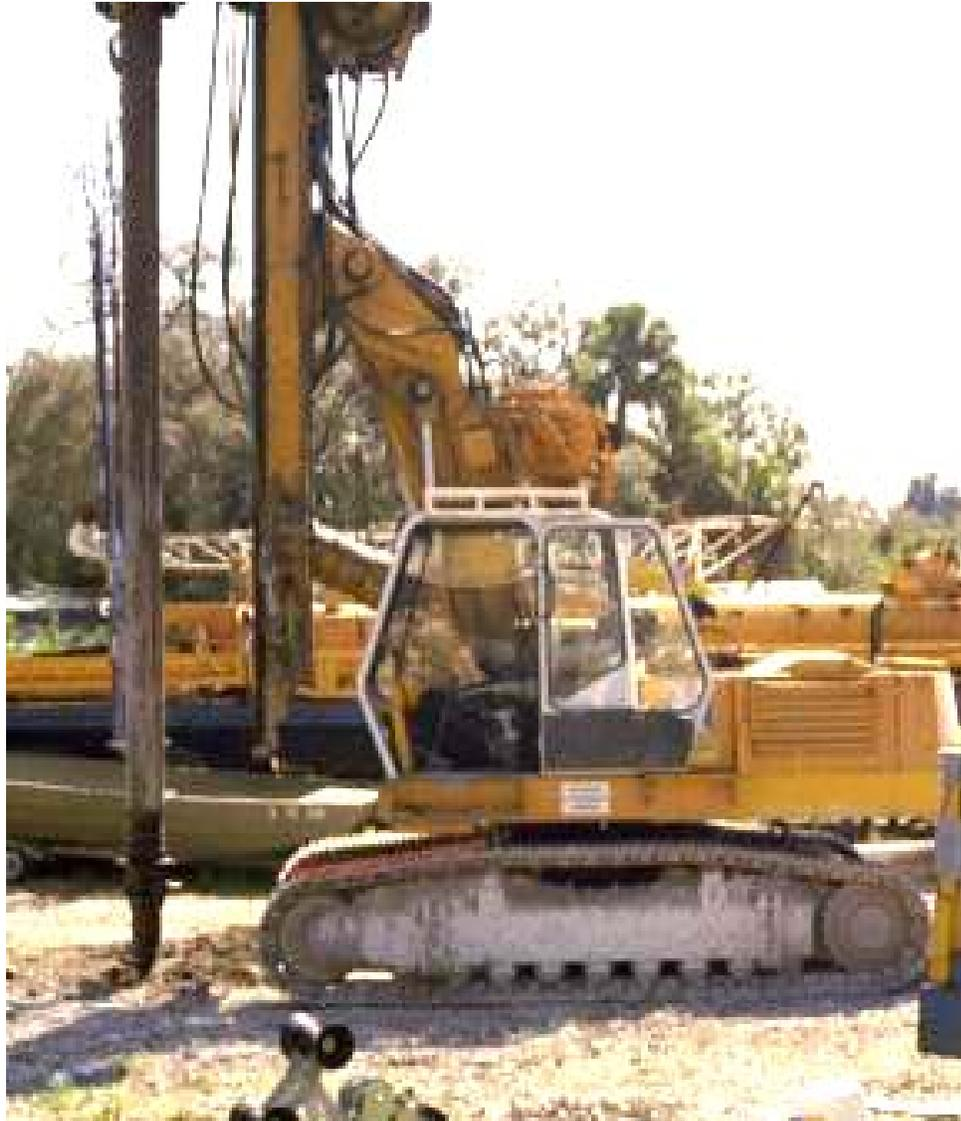
Figure 4-31. Site II excavation with a Bauer BG-7 drill rig.
