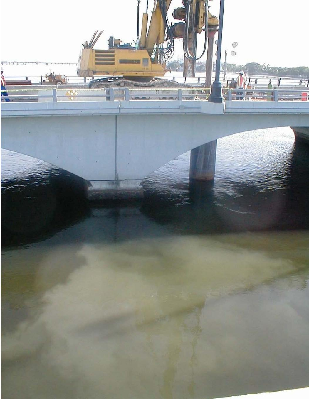
Figure 4-39. Slurry plume as Delmag drill rig excavates Site III LT-2.
