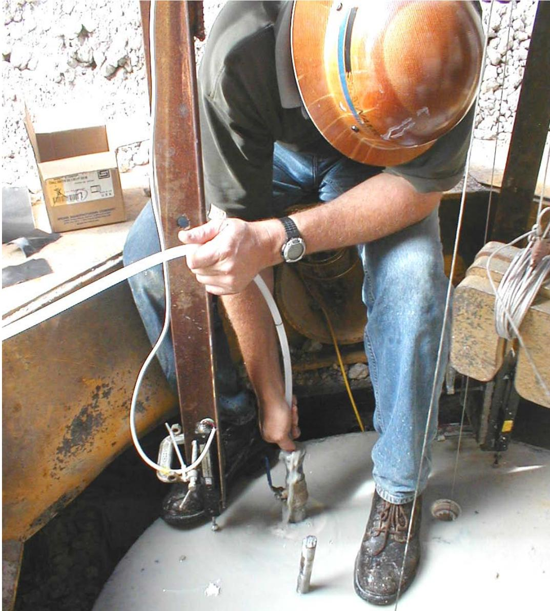
Figure 4-48. Grout lines flushed on Site III LT-2.
