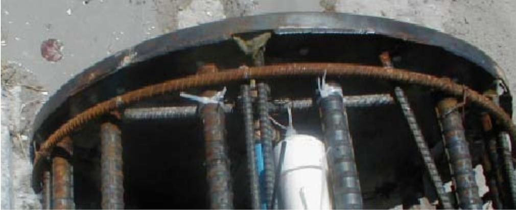
Figure 4-27. Site III tension telltale installed.
