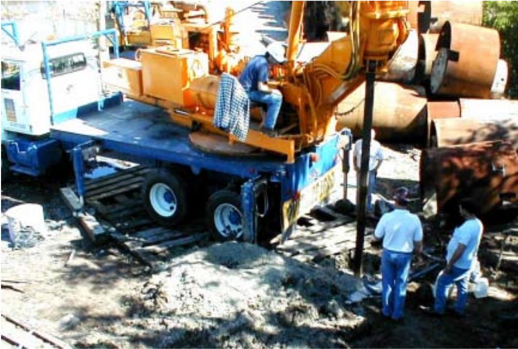
Figure 4-30. Site I excavation with a Texoma 700 drill rig.
