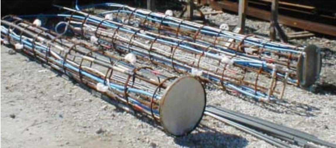
Figure 4-29. Sites I and II completed reinforcing cages with grouting apparatuses.
