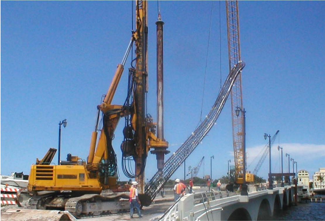
Figure 4-41. Kobelco crane lifting Site III LT-2 Cage.
