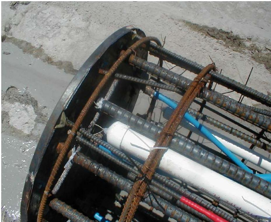
Figure 4-38. Site III LT-2 completed cage tip.
