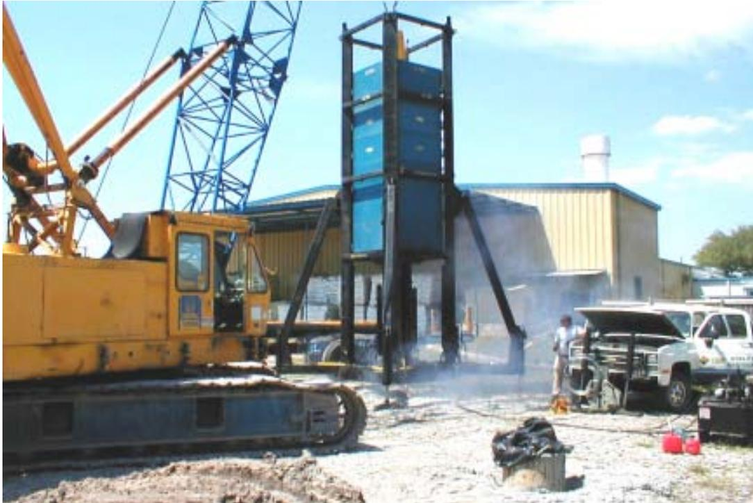
Figure 4-47. Statnamic load test in progress at Site II.
