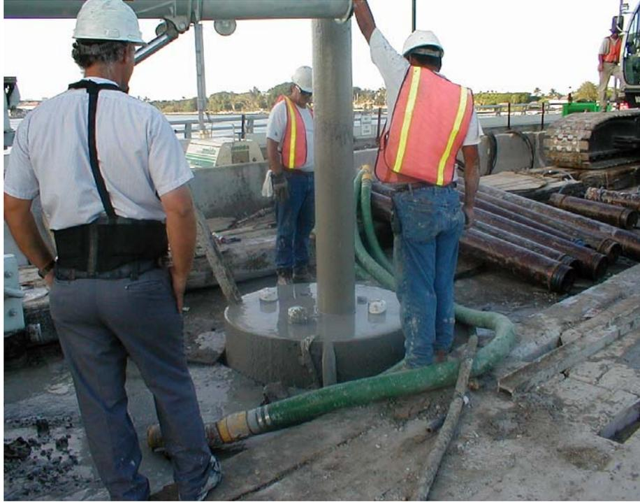
Figure 4-43. Concrete placement for Site III LT-2.
