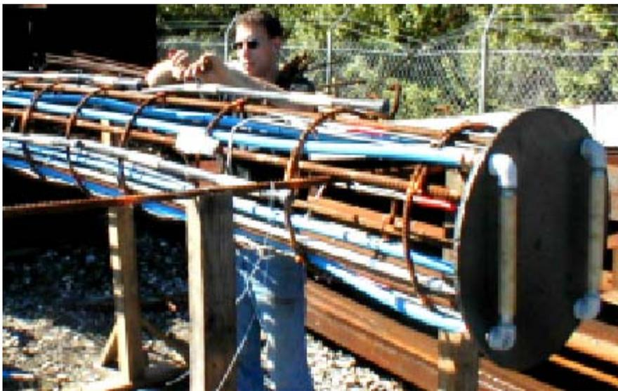
Figure 4-25. Skin grouting Sleeve-ports Tied into Cage (Site II).
