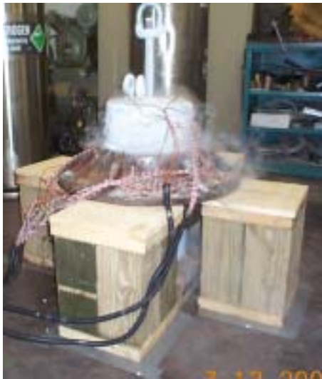
Figure 7.9 Completed Step 2 of AP1 with the cold trunnion inserted into the hub.
