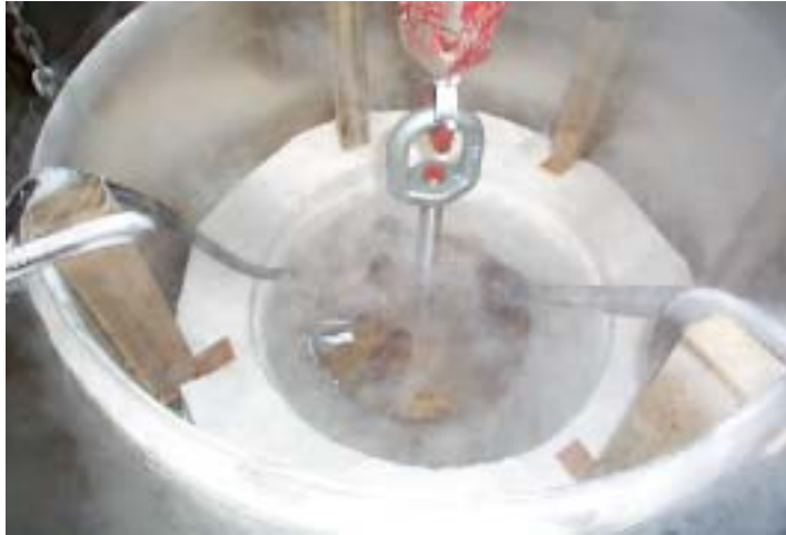
Figure 7.3 Trunnion immersed in liquid nitrogen (Step 1 of AP1).
