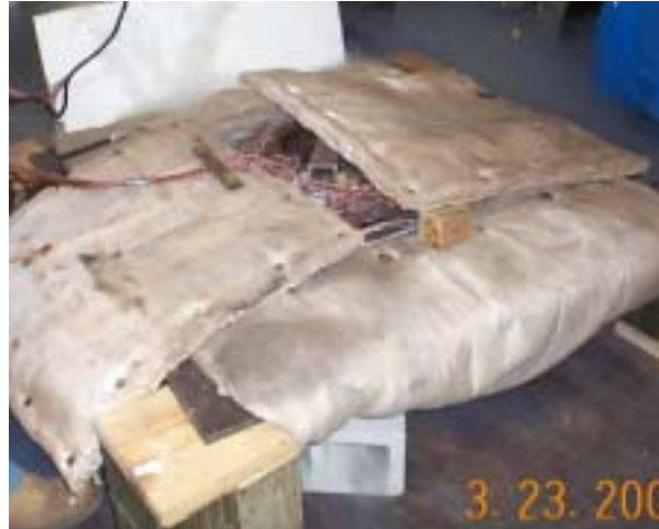
Figure 7.22 Induction heating coils for heating the hub-girder.
